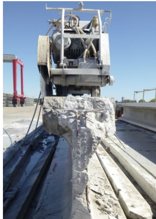
FIGURE 6-11: FINISHED SAW CUTS FOR CUT FLANGE GIRDER
