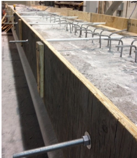
FIGURE 6-25: TIES WITH PVC PIPE SPACED 3FT APART TO HOLD FORM SIDES
