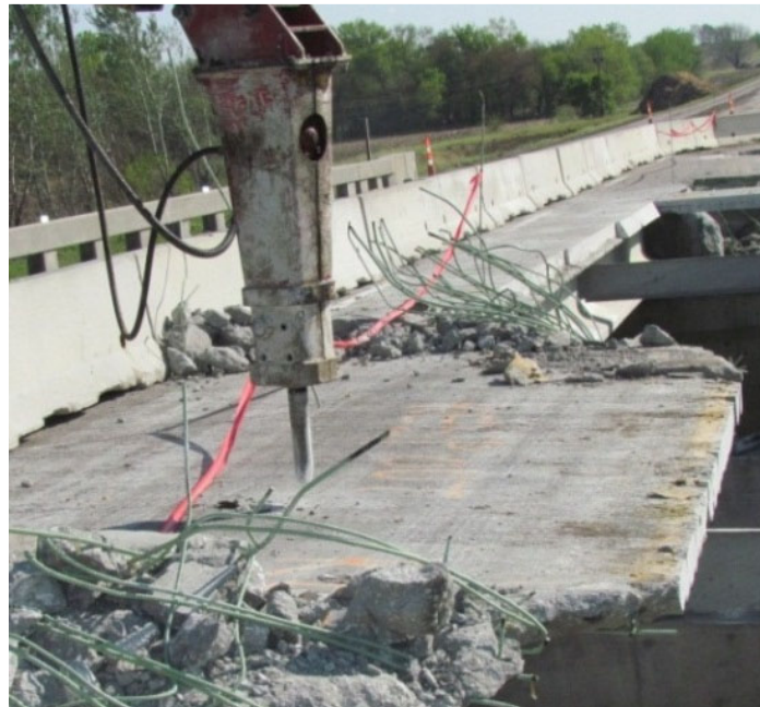
FIGURE 3-14: JACK HAMMERING THE DECK USING BACKHOE
