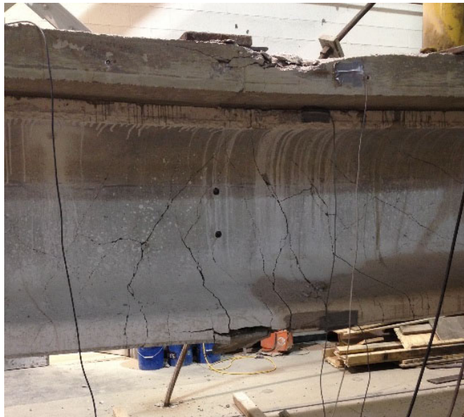
FIGURE 6-38: CUT FLANGE GIRDER FAILURE MODE
