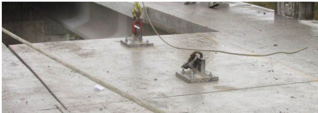
FIGURE 3-7: LIFTING ONE SIDE OF THE PANEL TO BREAK IT LOOSE
