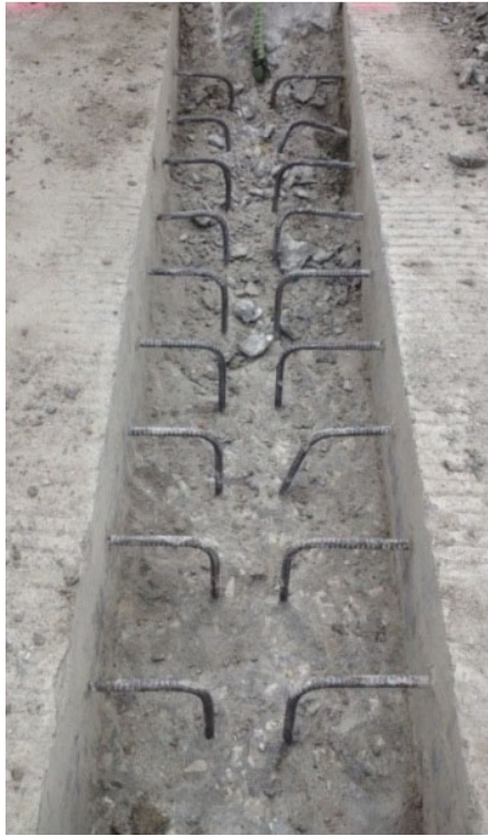
FIGURE 3-16: 14" WIDE X 5" LONG FULL DEPTH JACK HAMMERED STRIP
