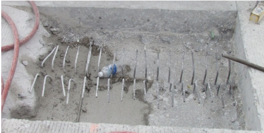
FIGURE 3-17: THE 4'10" X 3'2" JACK HAMMERED STRIP
