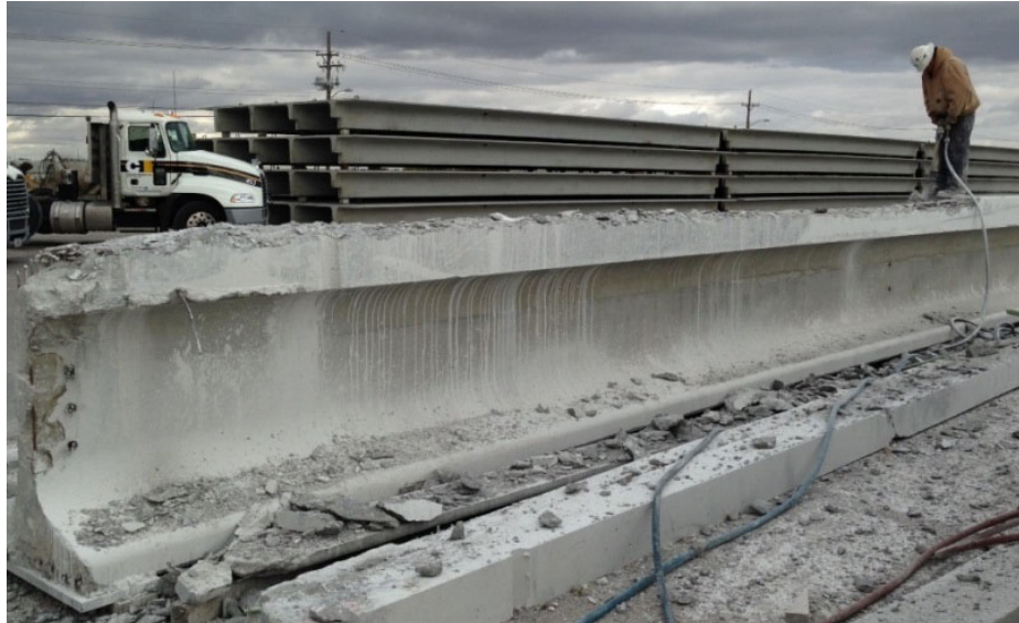
FIGURE 6-15: JACK HAMMERING DOWN TO STIRRUPS
