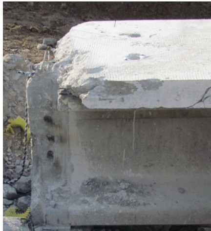
FIGURE 6-2: VIEW OF GIRDER END AND LOCATION OF TWO CONCRETE CORES
