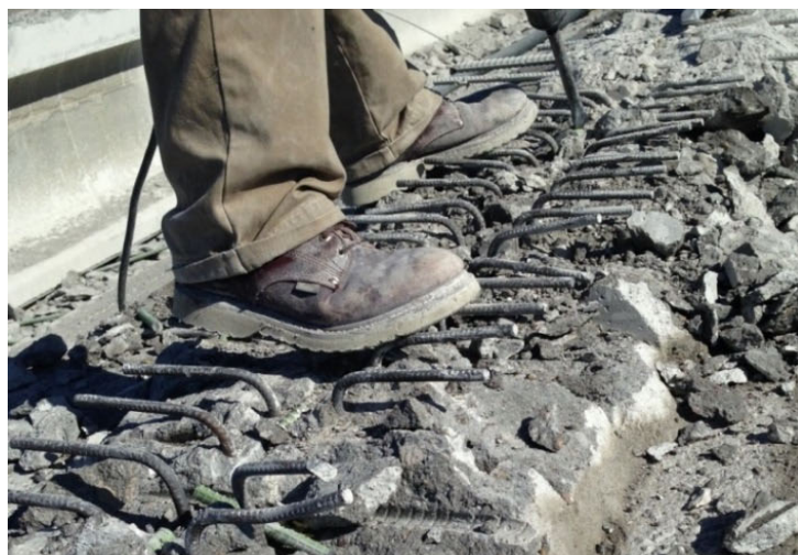
FIGURE 6-21: 1-2 IN. OF SPACE UNDERNEATH STIRRUP LEGS
