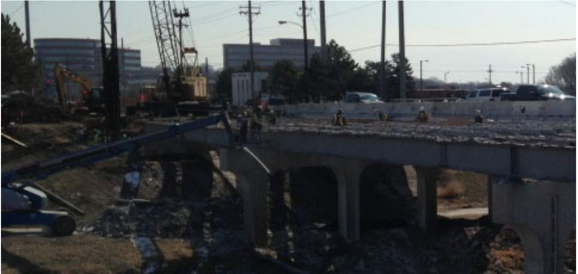
FIGURE 3-30: WORKERS USING HAND CHIPPERS TO REMOVE CONCRETE AROUND SHEAR STUDS
