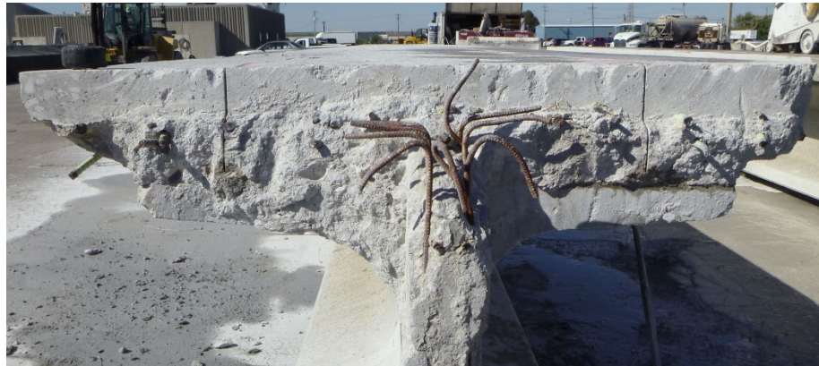
FIGURE 6-8: FINISHED SAW CUTS (BEFORE END DECK SECTIONS WERE REMOVED)
