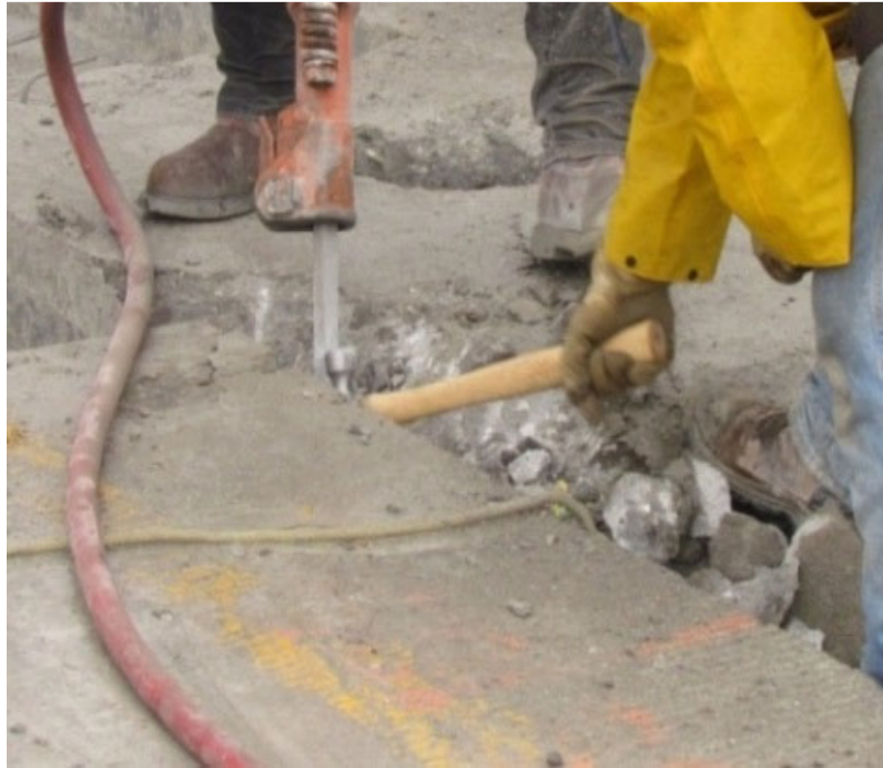
FIGURE 3-9: JACK HAMMERING THE DECK ATTACHED TO THE PANEL HAUNCH
