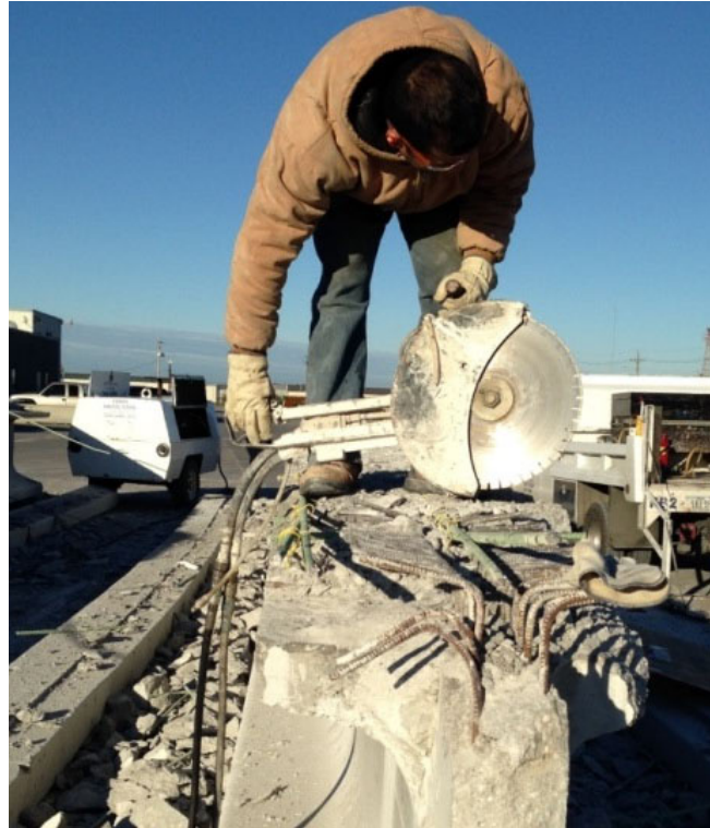
FIGURE 6-18: TRANSVERSE SAW CUTTING EVERY 5 IN.
