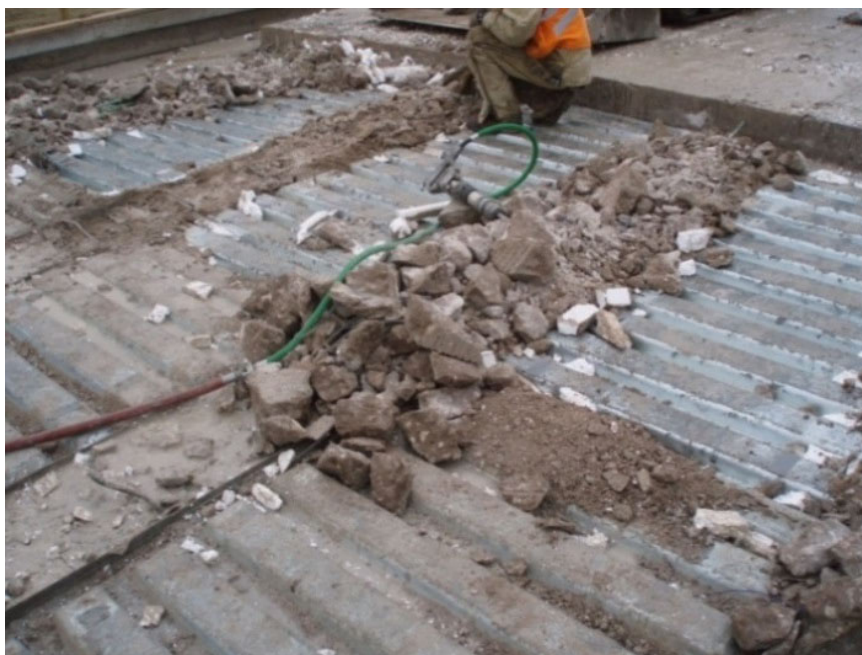
FIGURE 3-22: JACK HAMMERING ABOVE THE GIRDERS
