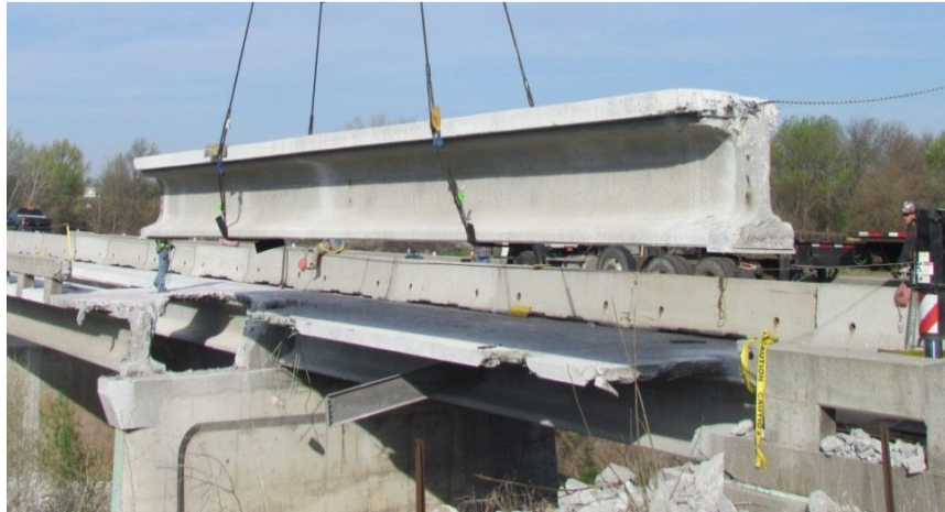
FIGURE 6-1: CAMP CREEK GIRDERS LIFTED USING STRAPS
