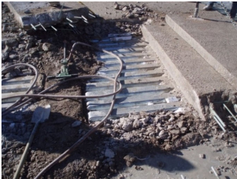
FIGURE 3-21: DECK PANEL LIFTED FROM STAY-IN-PLACE FORMS BETWEEN GIRDERS
