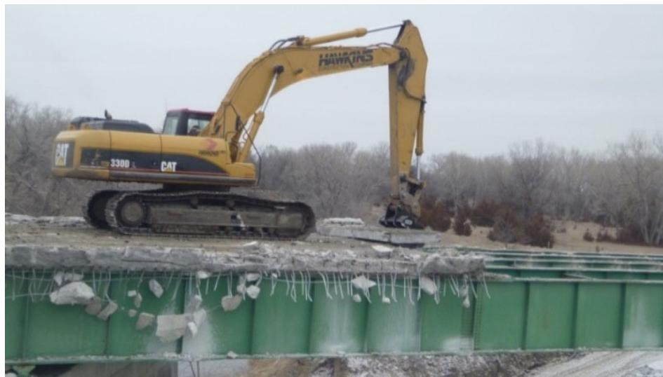
FIGURE 3-26: SLAB CRAB LIFTING DECK SLAB FROM WEST TO EAST
