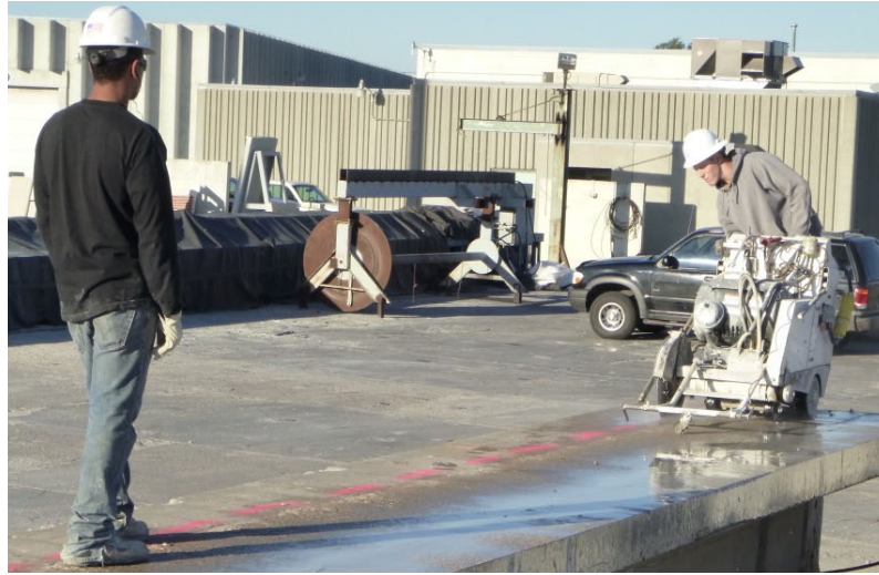
FIGURE 6-7: WORKERS MAKING THREE PASSES FOR EACH SAW CUT LOCATION
