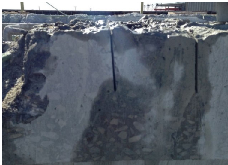
FIGURE 6-19: DEPTH OF SAW CUTS ABOUT 4 IN.; 1 IN. FROM TOP FLANGE
