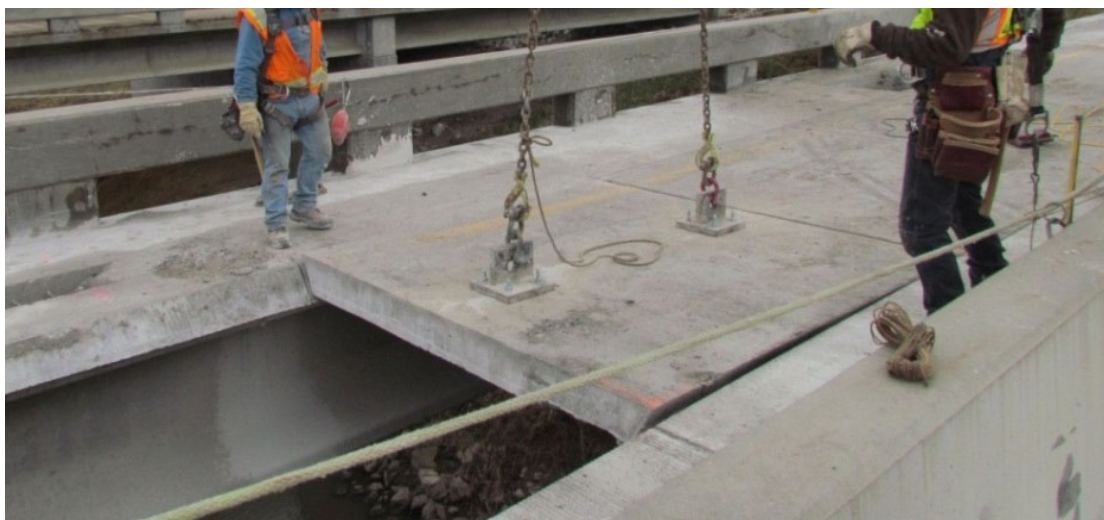
FIGURE 3-11: LIFTING THE SLOPPED CUT PANEL
