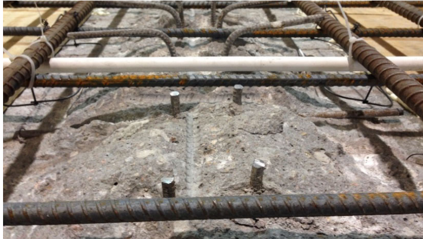
FIGURE 6-28: CUT SHEAR CONNECTORS IN PARTIALLY REMOVED SECTION
