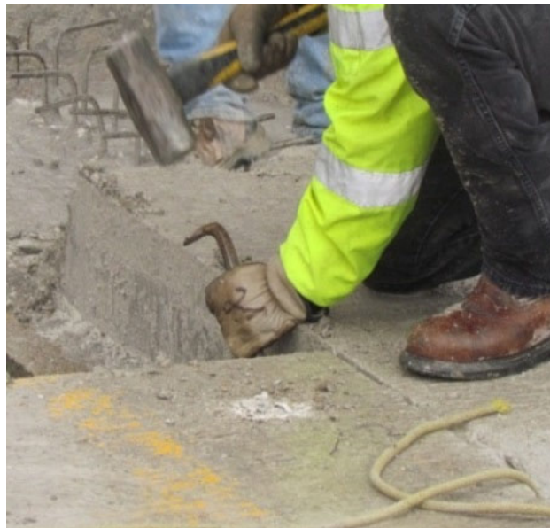
FIGURE 3-8: BREAKING PANEL FROM DECK USING A HAMMER AND A CHISEL
