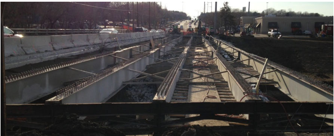
FIGURE 3-31: VIEW LOOKING WEST AFTER COMPLETED DECK REMOVAL
