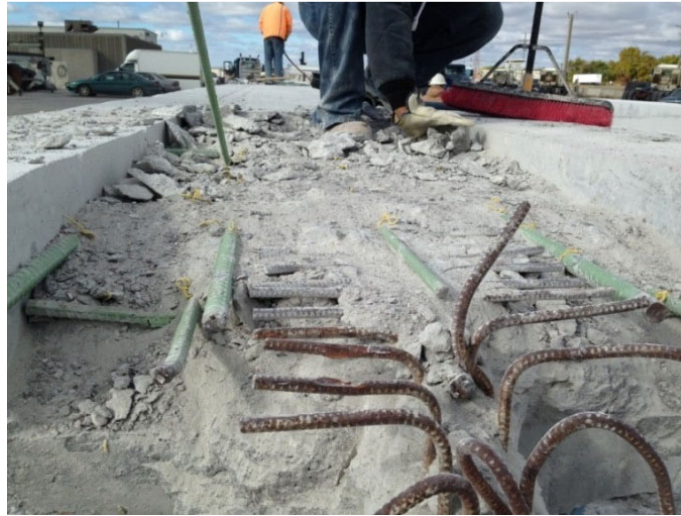
FIGURE 6-14: DIFFICULT REMOVING CONCRETE UNDER LONGITUDENAL BARS
