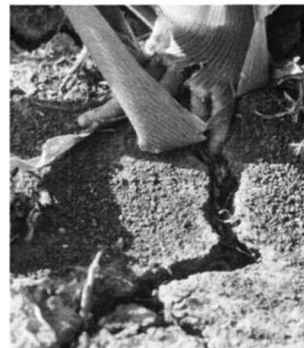
Cracks, many much deeper than these, are typical in fields and pastures across drought-stricken areas of the state.
