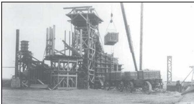
**Construction of Minatare Dam in western Nebraska, like many early Reclamation projects, included having to elevate skips containing gravel into a hopper that screened the gravel. This photo dates to November, 1912. For perspective, that's little more than seven months after the ocean liner RMS TITANIC struck an iceberg and sank in the North Atlantic (USBR photo).**
