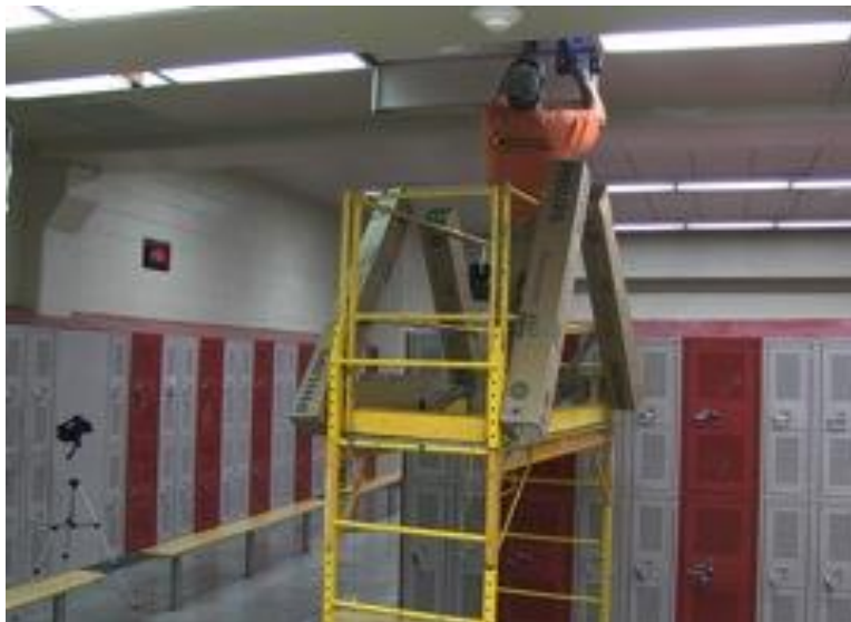
Figure 5.7: Ballast Cover Closure
