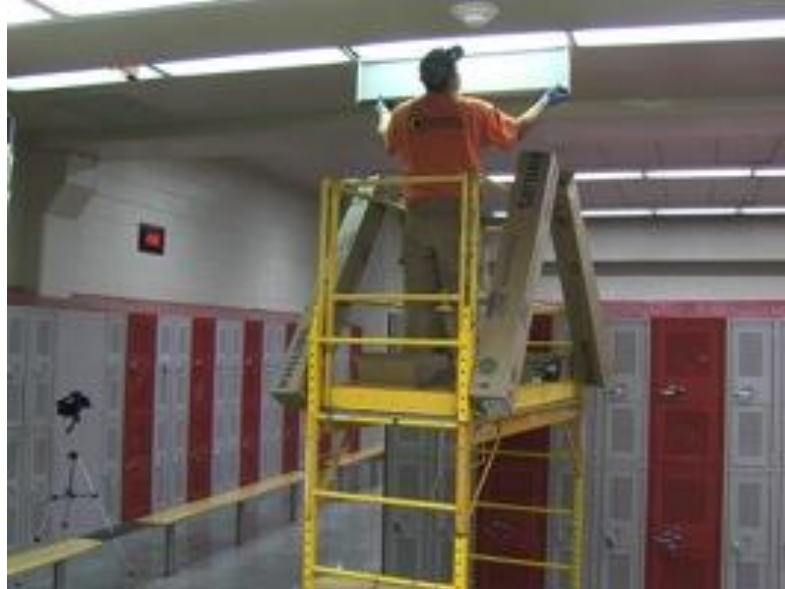
Figure 5.2: Glass Frame Removal
