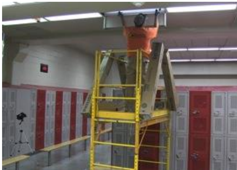
Figure 5.8: New Bulb (T8) Installation
