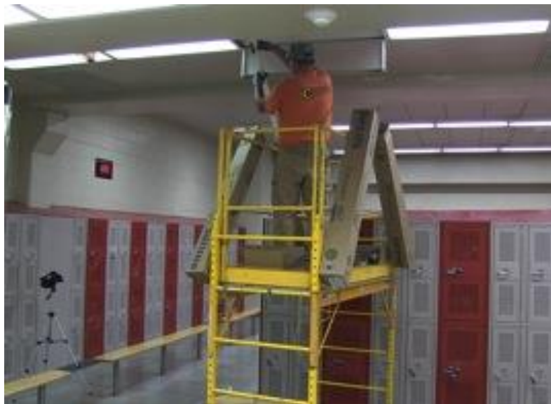
Figure 5.3: Old Bulb (T12) Removal
