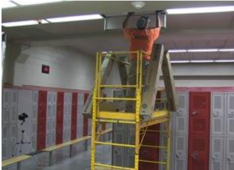
Figure 5.6: New Ballast Installation
