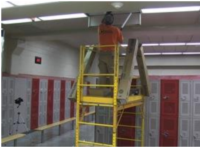
Figure 5.5: Old Ballast Removal
