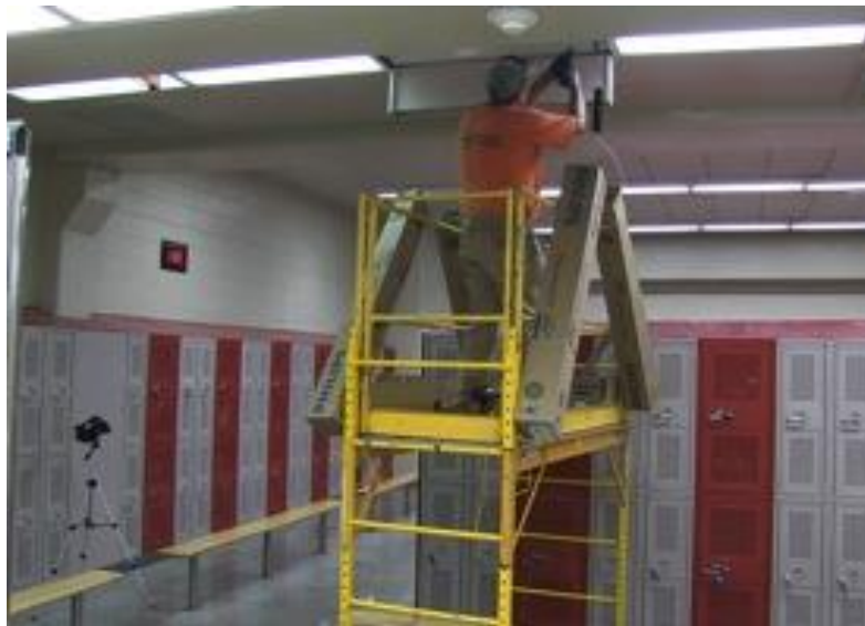
Figure 5.4: Ballast Cover Removal
