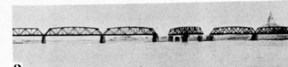
1. A. PONTON BRIDGE. B. SIMPLE TRUSS, MULTIPLE SPAN BRIDGE. C. PONTON BRIDGE. 2. STEEL TRUSS, ARCH BRIDGE. 3. SIMPLE TRUSS, MULTIPLE SPAN BRIDGE WITH SWING DRAWBRIDGE. 4. LARGE, SEGMENTAL, SINGLE SPAN ARCH. 5. MULTIPLE SPAN, ARCH-SUSPENSION BRIDGE. 6. VERTICAL: SUSPENSION BRIDGE 7. VERTICAL: ARCH-SUSPENSION BRIDGE
