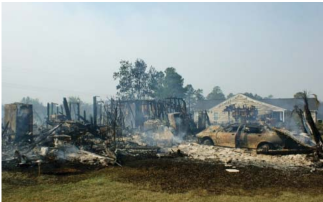
A home smolders after the April 2009 Highway 31 Fire in South Carolina.
