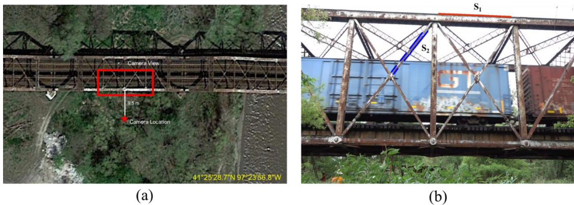
Figure 10 (a) Camera Location; (b) Image view of the railway bridge along with active pixels extracted at structure S_1 (in red) and S_2 (in blue)
