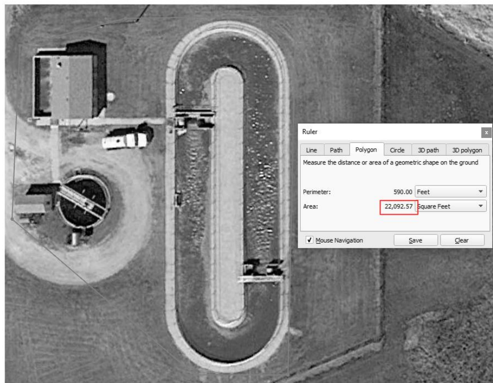
Figure D12. Basset Aerial View
