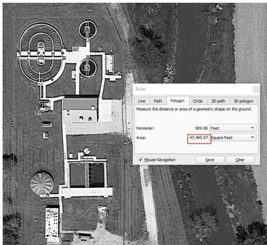
Figure D13. Albion Aerial View
