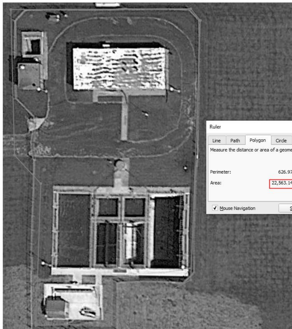
Figure D18. Syracuse Aerial View
