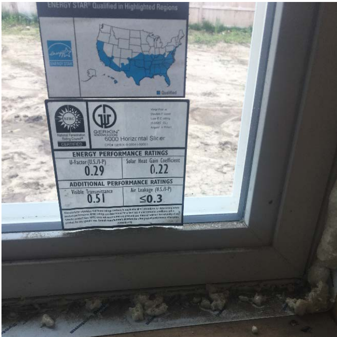
Figure 3.4 Window U-factor Verification
