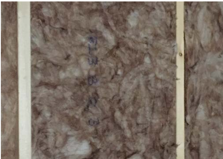
Figure 3.2 Exterior Wall Fiberglass Batt Insulation Verification
