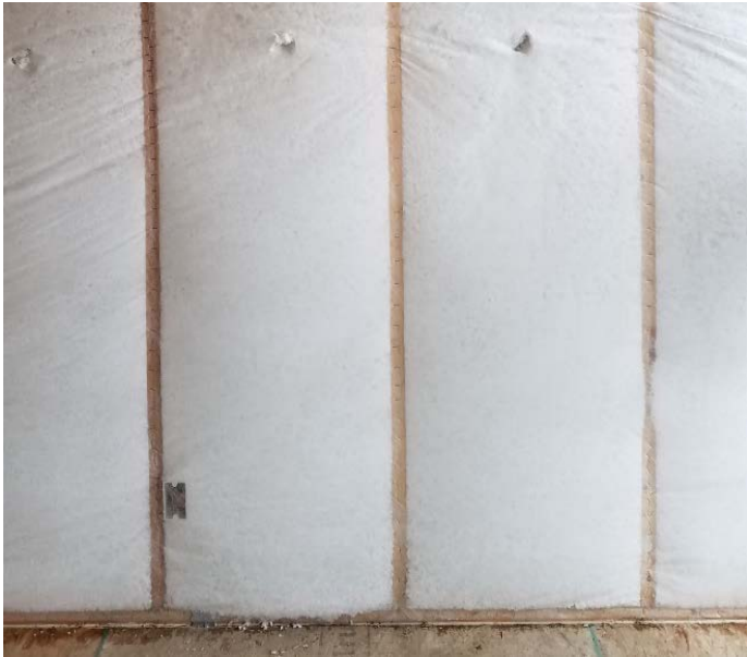
Figure 3.3 Exterior Wall Blown-in Insulation Verification
