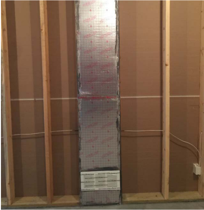
Figure 3.5 Duct Sealing Verification
