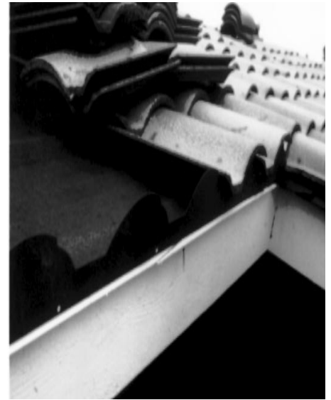
Fig. 25. "Bird stop" shaped metal for tile roofs to prevent rodent and bird entry.
