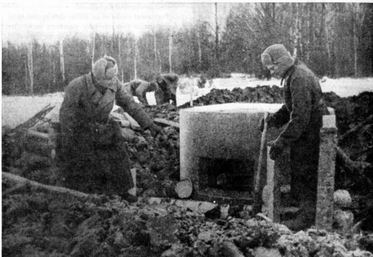
Figure 28.—Pre-fabricated pillbox.
