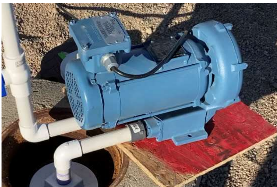
Figure 5.2: Gas Capture System
