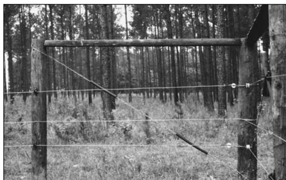
Energized high tensile wire fence will withstand falling debris. Strategically locate power switches to improve pasture access and diagnosing power failures.
