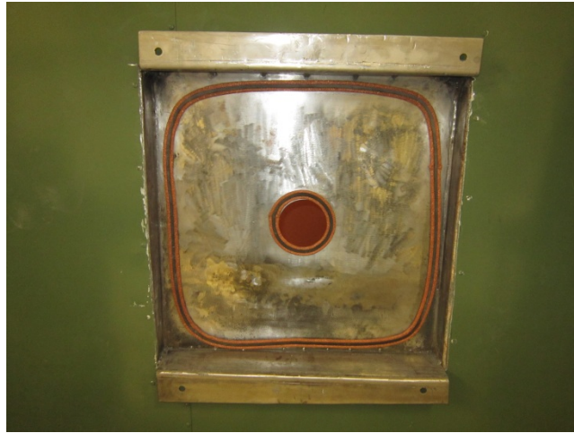
Figure 3-18: Gaskets on RF shelter test port
