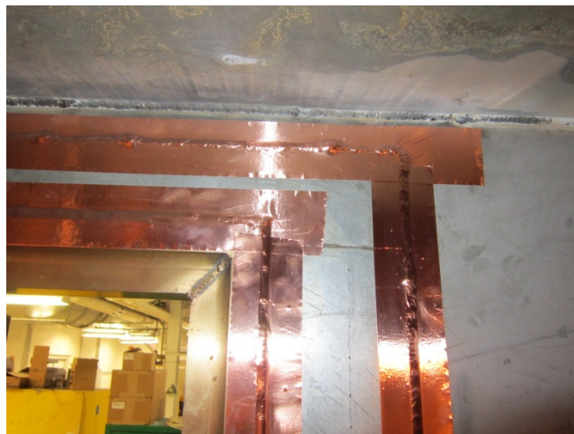
Figure 3-11: Copper tape used to seal RF leaks in shelter
