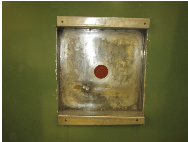
Figure 3-12: Square hole cut in shelter skin with mounting shelves installed and test port
