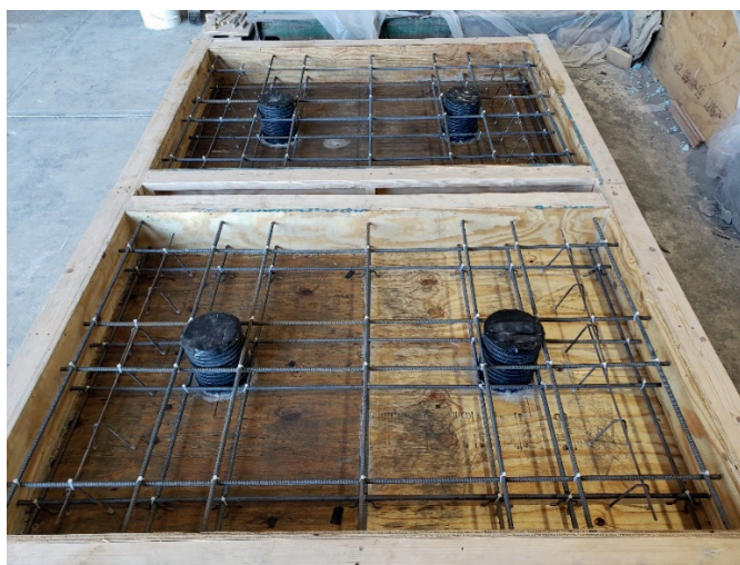
Figure 6.31. Shear Pockets Forming and Slab Reinforcement Details.
