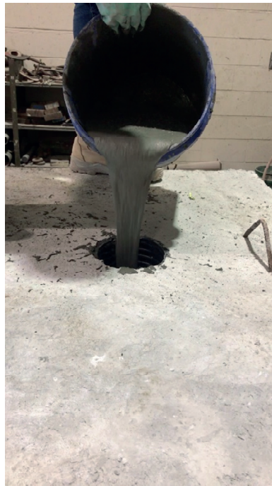
Figure 6.34. UHPC Casting for UHPC#2 Specimen.
