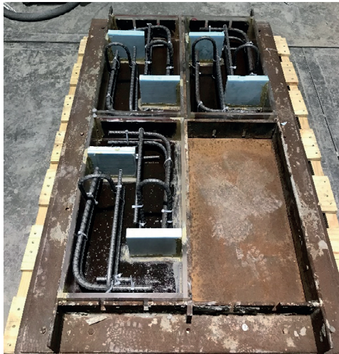
Figure 6.5. L-Shape Push-off Specimen Preparation.
