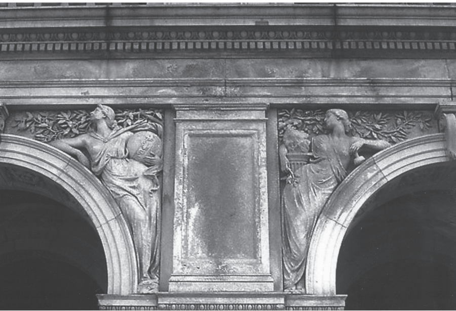
1. Spandrels at the Library of Congress Building in Washington DC. Photo by Einar Einarsson Kvaran. Use authorized under the GNU Free Documentation License.
