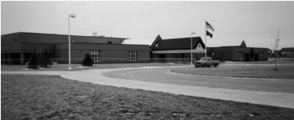
Fig. 2.1. Maxey Elementary School, one of four identical schools in Lincoln Nebraska, served by geothermal heat pumps.
