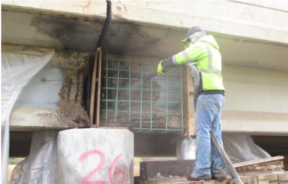
Figure 4: Reinforced concrete encasement of a deteriorated bridge girder end, courtesy of MN/RC 2018-07 Report
