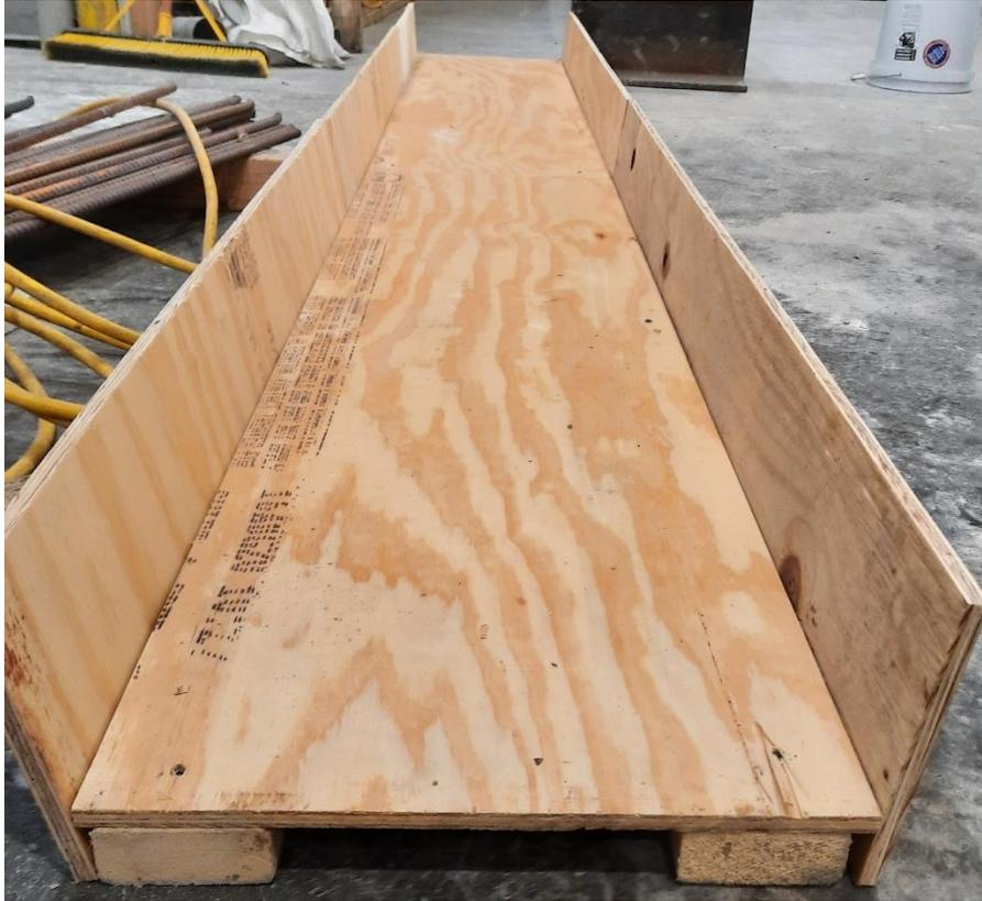
Figure 105: Flexural strengthening procedure, step 4: assembling formwork
