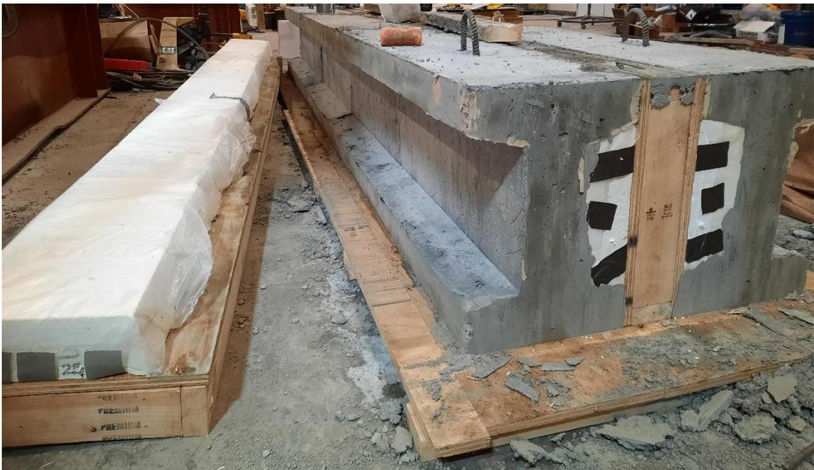
Figure 101: Stripping formwork of two CC beams
