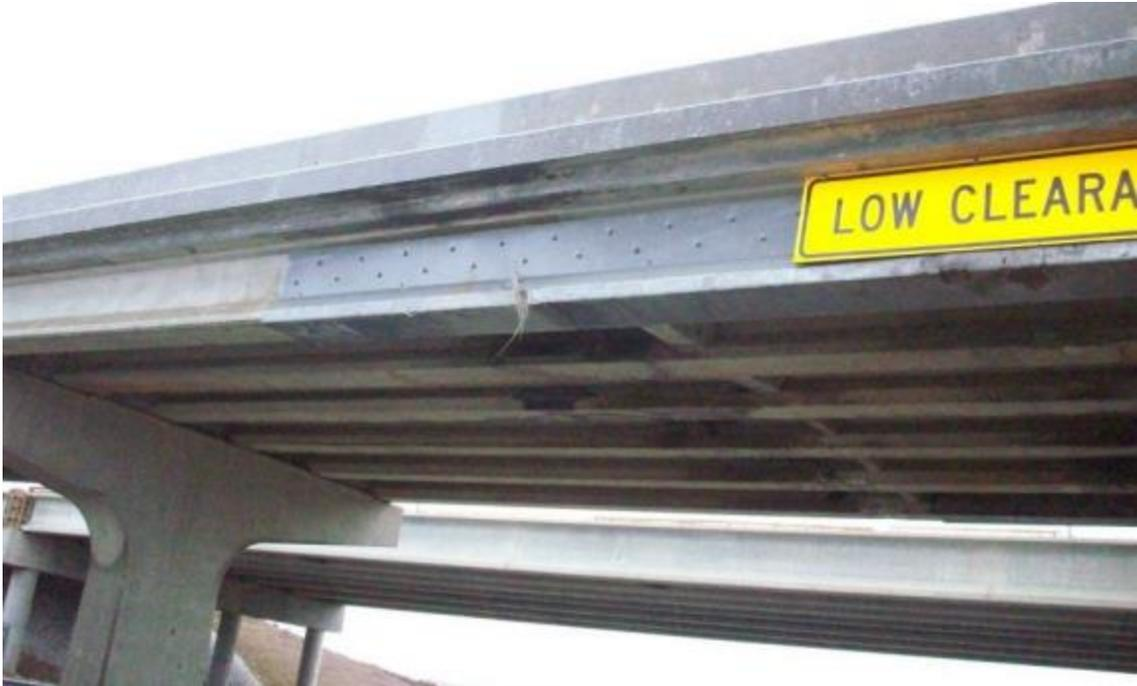
Figure 7: Grouted steel encasement of a bridge girder, courtesy of Iowa Dot, 2014
