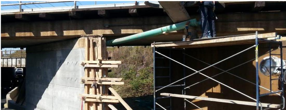
Figure 11: Casting UHPC using a chute for a thin jacket for a bridge pier from the top of formwork, courtesy from Ductal website and Doiron, 2017
