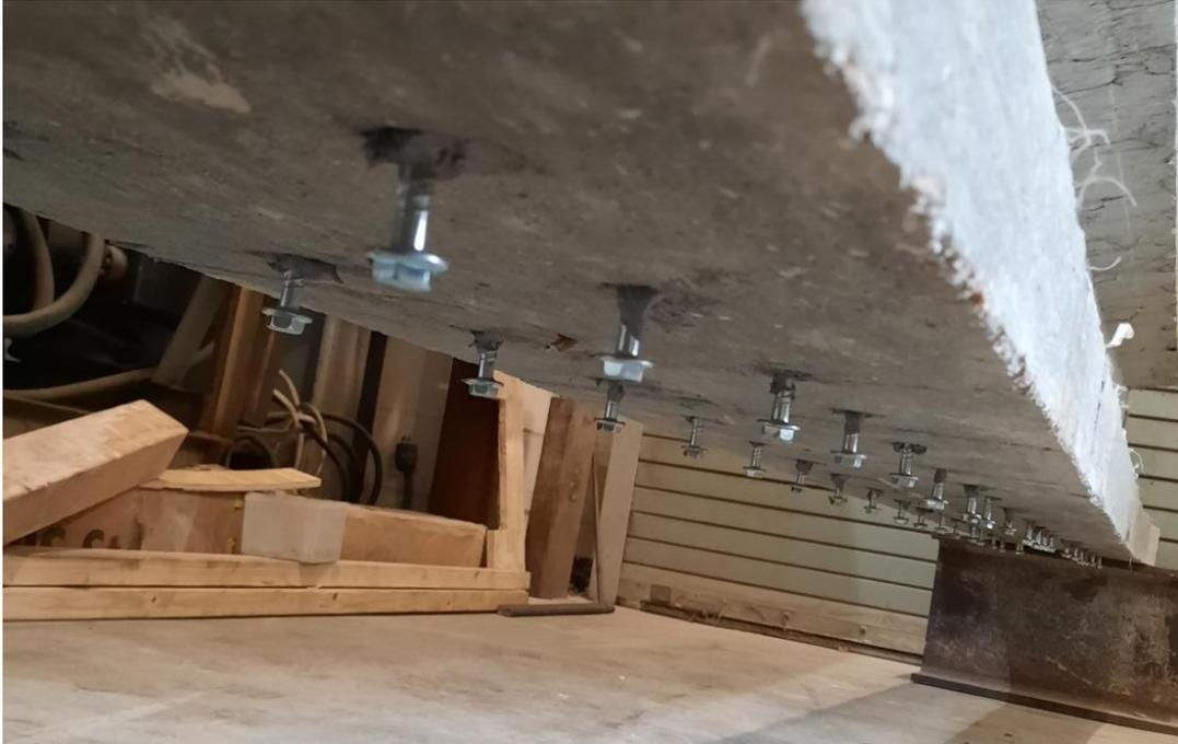
Figure 103: Flexural strengthening procedure, step 2: installing anchors
