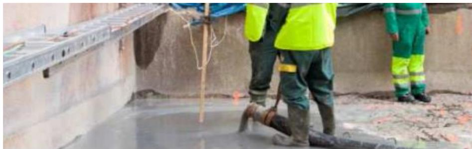
Figure 17: Pumping UHPC to repair the Caderousse Dam slab, courtesy of Guingot et al., 2013
