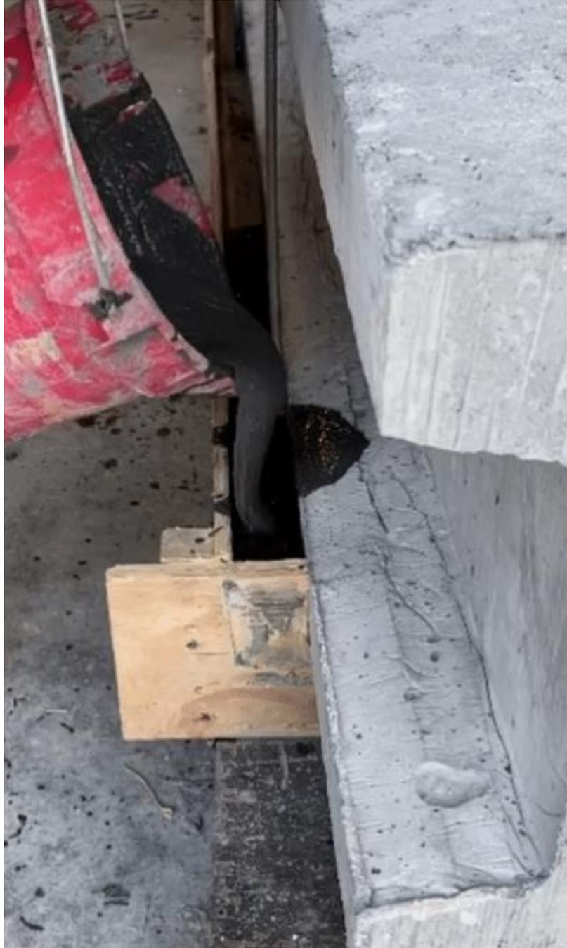
Figure 107: Flexural strengthening procedure, step 6: pouring UHPC
