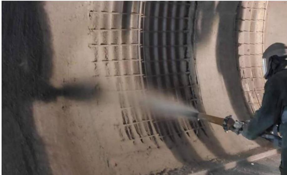
Figure 18: UHPC shotcrete to strengthen and renovate a deteriorated metal culvert, courtesy of Ductal website
