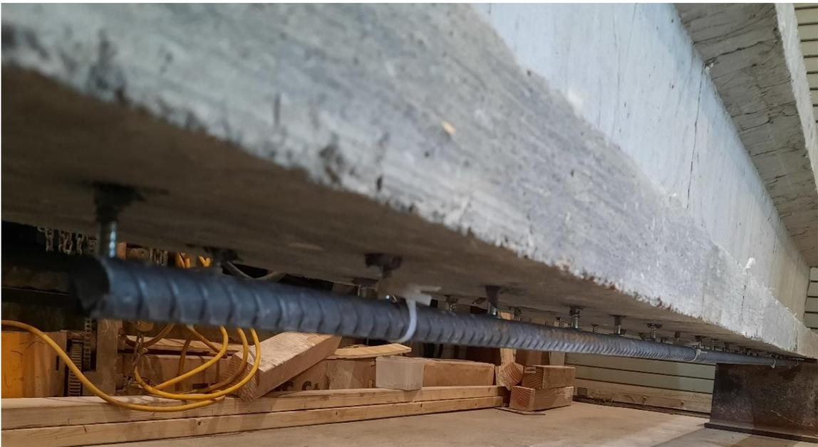
Figure 104: Flexural strengthening procedure, step 3: installing additional reinforcement
