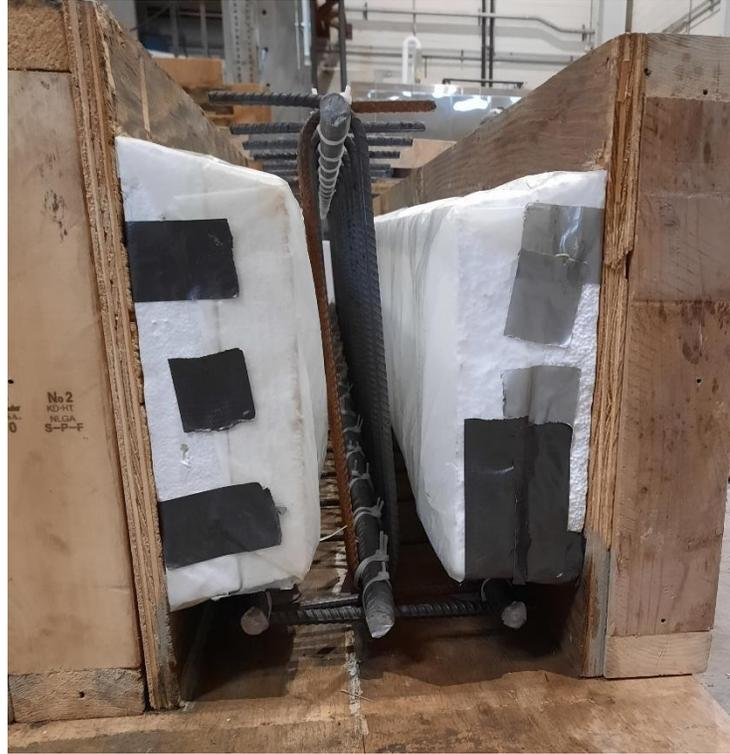
Figure 100: Formwork and reinforcement of one of the CC beams
