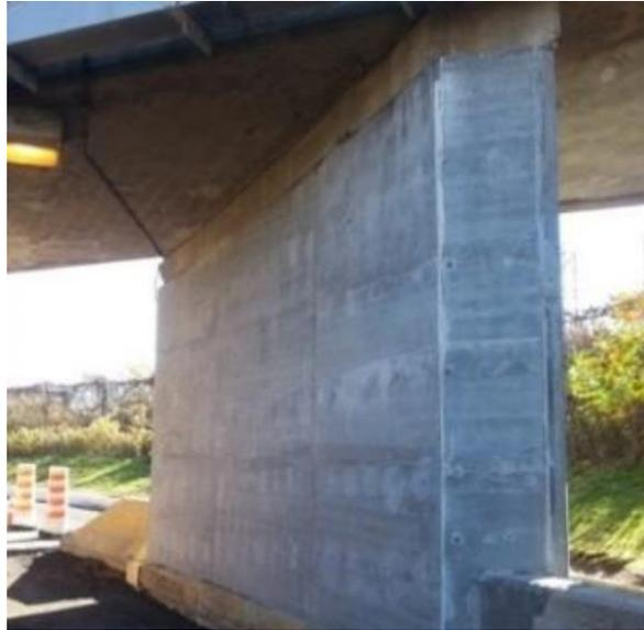
Figure 12: UHPC jacket over the bridge pier, courtesy of Doiron, 2017
