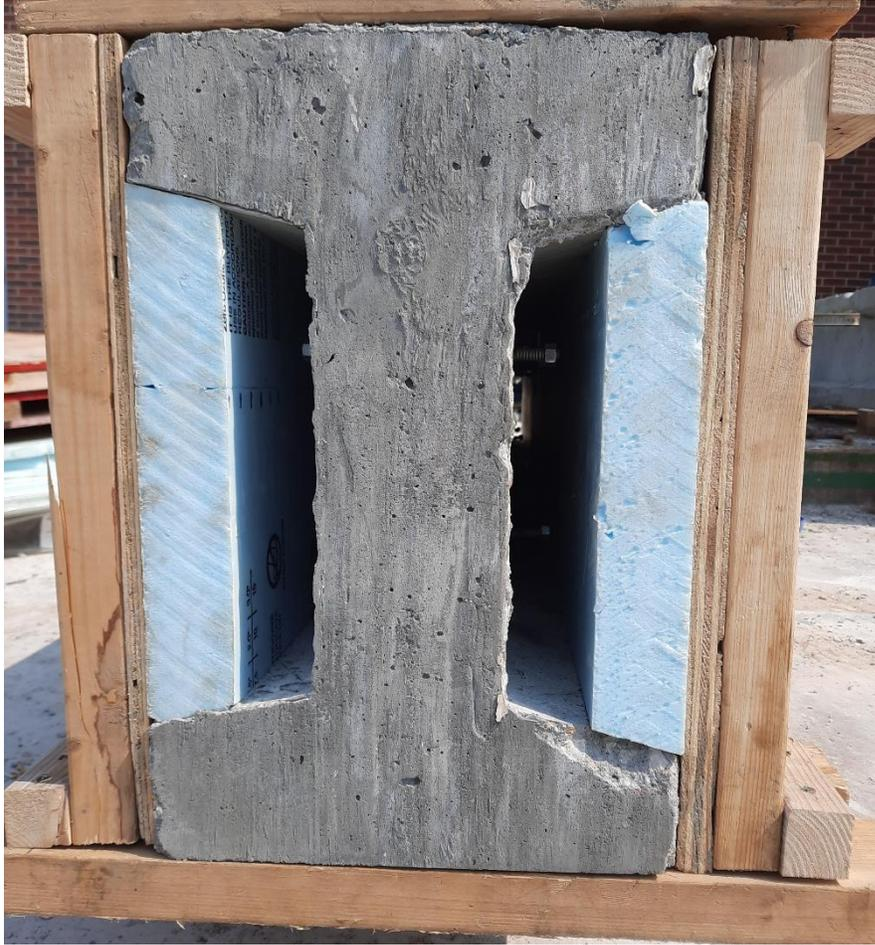
Figure 134: Shear strengthening procedure, step 4: installing formwork
