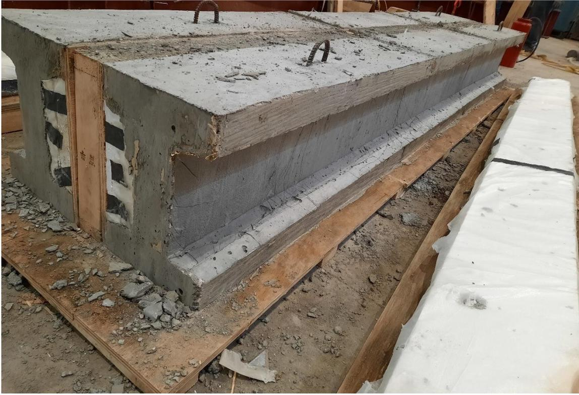
Figure 131: Stripping formwork of two CC beams
