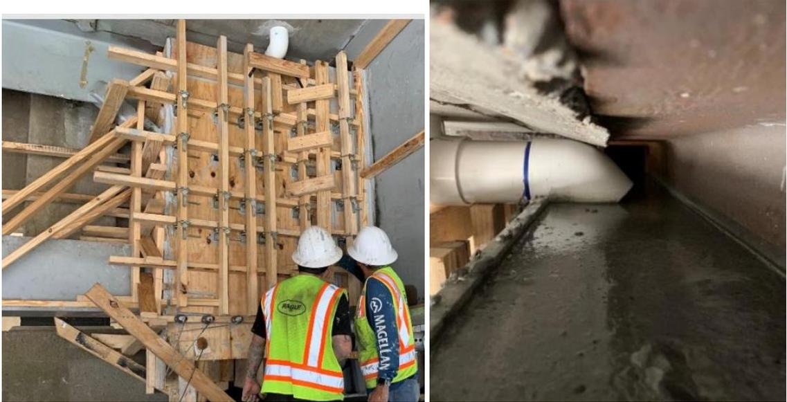
Figure 9: Pouring UHPC from the top of a concrete bridge deck using pipes for strengthening a steel bridge girder, courtesy of Fan, 2020
