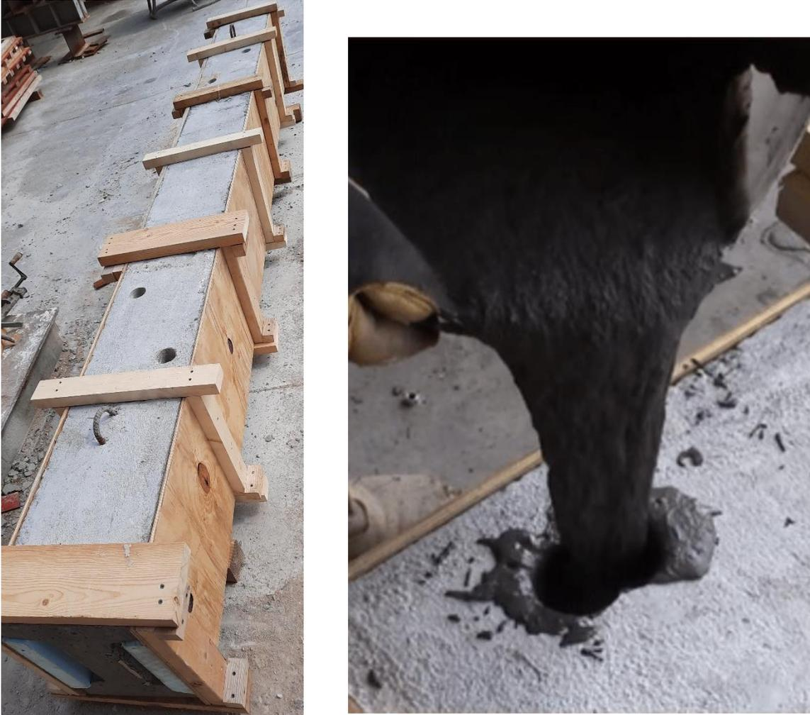
Figure 135: Shear strengthening procedure, step 5 (left): fixing formwork, step 6 (right): pouring UHPC
