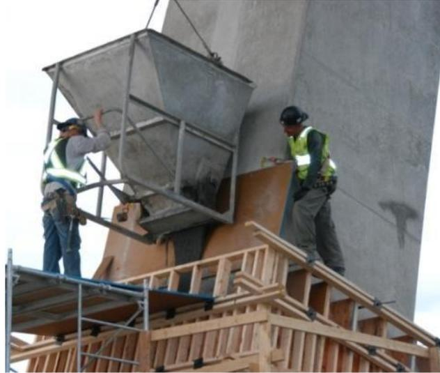
Figure 13: Casting a 9-inch thick UHPC jacket around a bridge pier using a hopper, courtesy of Doiron, 2017
