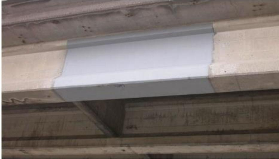
Figure 5: FRP Wrapped Repair, courtesy of Iowa Dot, 2014
