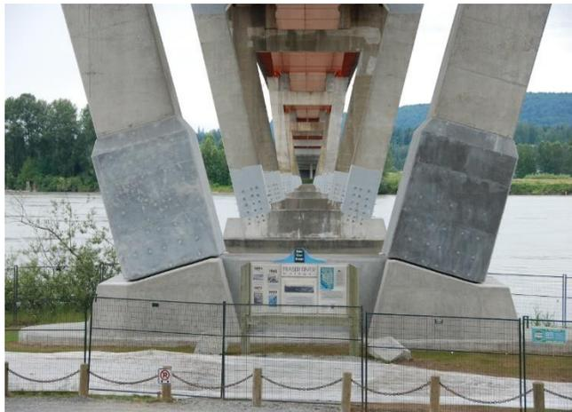
Figure 14: Seismic strengthening with UHPC jackets around bridge piers, courtesy of Doiron, 2017
