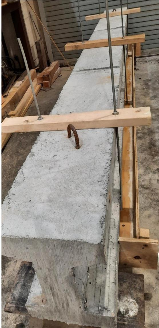
Figure 106: Flexural strengthening procedure, step 5: installing formwork
