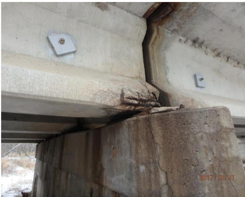
Figure 1: Deteriorated bridge girder end, Platte River South Bridge, courtesy of Nebraska Department of Transportation, Kodsy et al., 2020
