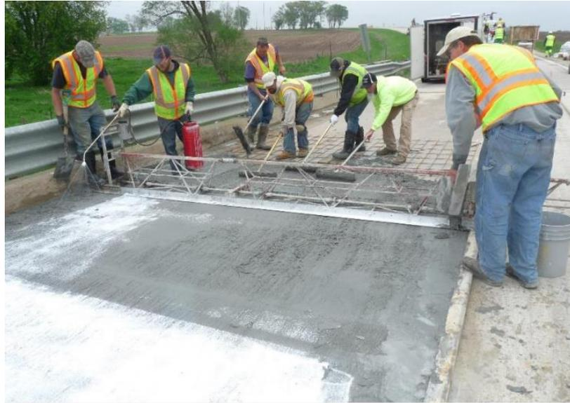
Figure 16: Placing UHPC deck overlay, Mud Creek Bridge, Iowa, Wibowo et al., 2018
