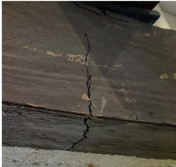
Figure 83: Flexure failure mode in the ribbed slab
