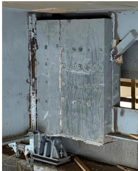
Figure 10: Strengthened girder end after stripping the forms, courtesy of Fan, 2020
