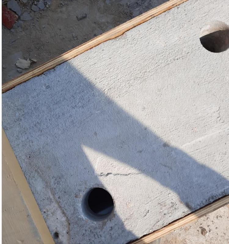
Figure 133: Shear strengthening procedure, step 3: drilling top flange openings
