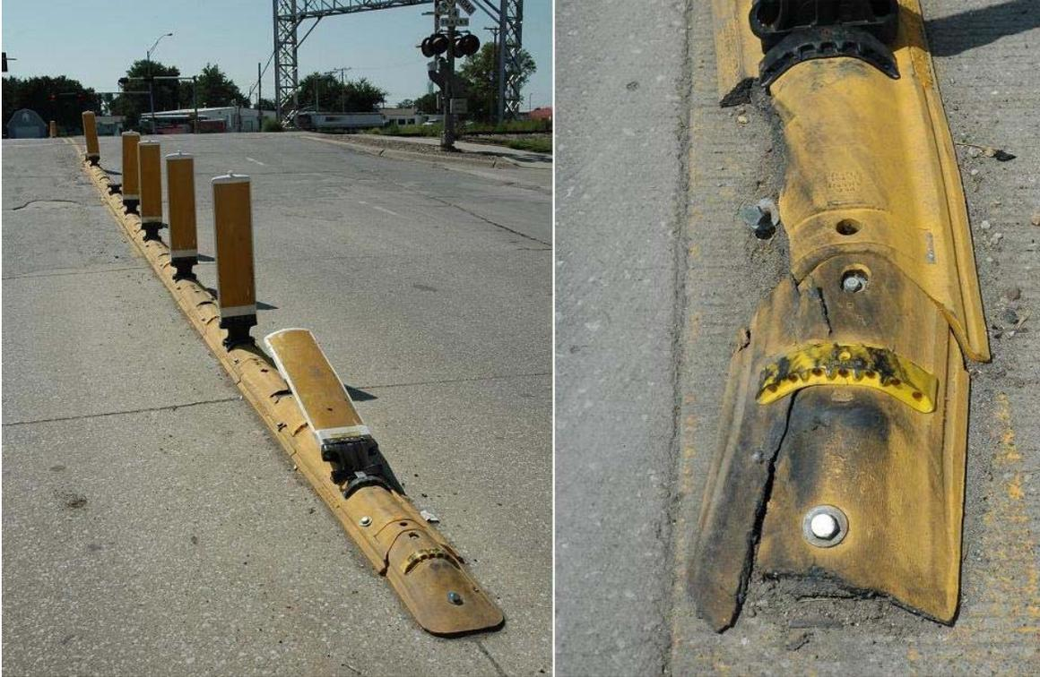
**Figure 4.1. Flattened and abused curbing due to overrunning trucks in Waverly**
