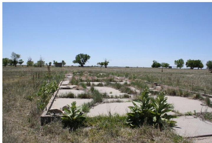
Figure 2.9: Building foundation at the camp.
