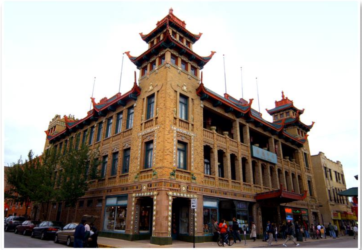
Figure 2.3 The Pui Tak Center in Chinatown, built in the Chinese style during the 1920s. Source: Chicago Chinatown Chamber of Commerce
