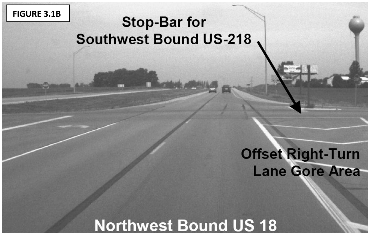
Figure 3.1 Site B, ORTL at West Junction of US-18 and US-218, Floyd, IA (6)
