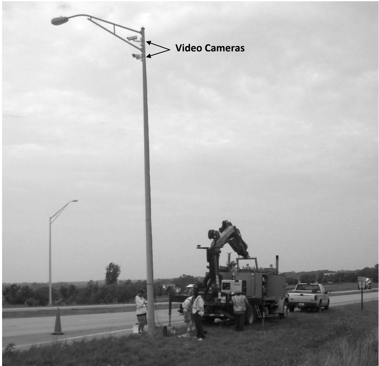
Figure 6.3 Field Assembly at Site 1 During Installation
