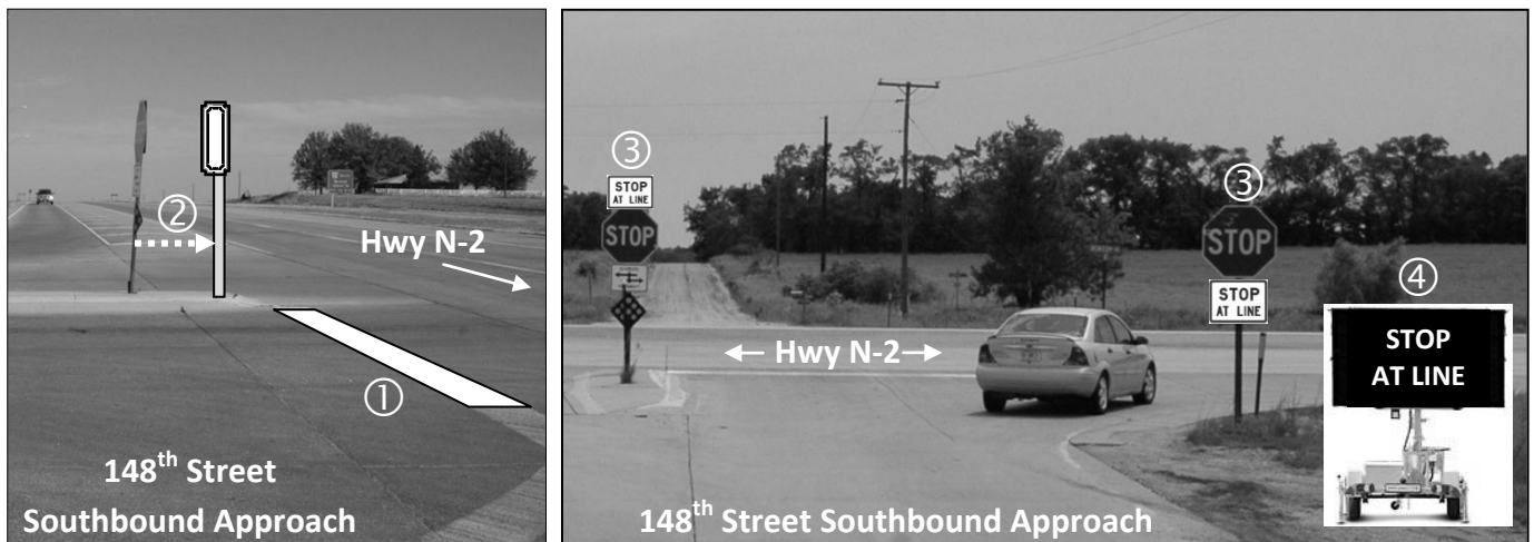
Figure 4.1 Preliminary Suggestions to Improve Stopped Driver Location Choice on Southbound Stopped Approach at 148 th Street.
