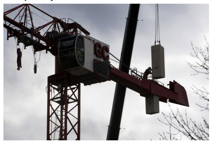
Workers construct a tower crane on the southeast corner of Ninth and O streets on March 30. The crane will be used to construct a 140-room Holiday Inn Express.
