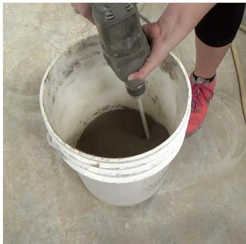
**Figure 3-1: Power mixing of soil-cement mixture**
