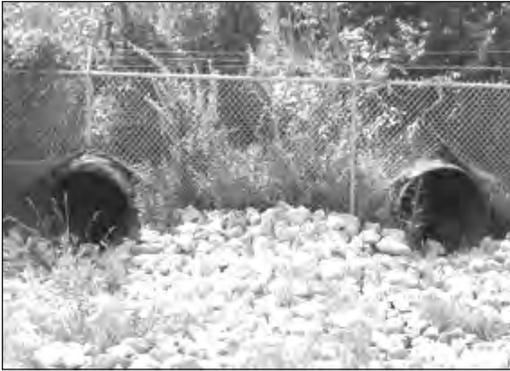
**FIGURE 1.** Culverts through a fence line can create large passageways for wildlife at airports. (Photo by J. E. Kubel)
