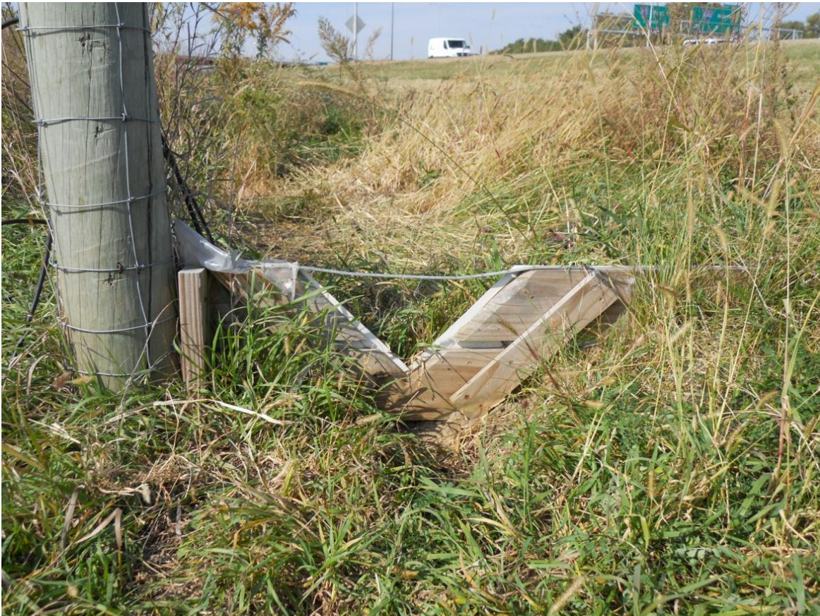
Figure 4.4 V-notch weir installed at site B
