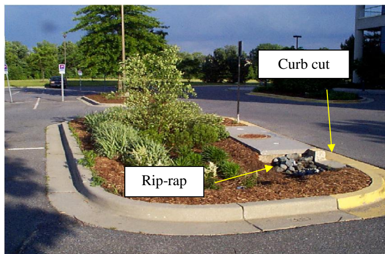
Figure 14 Curb cut inlet system (NCDENR 2007)
