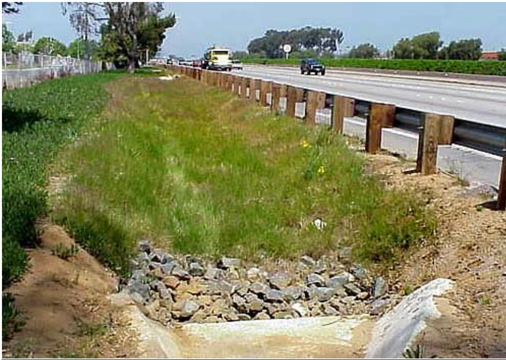
Figure 12.2 Roadside swale (CalTrans 2012)
