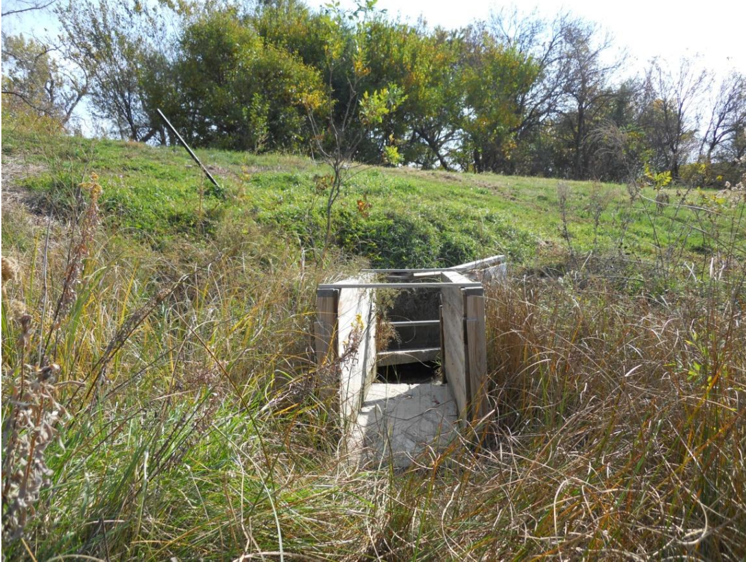
Figure 4.5 Rectangular flume installed at site E
