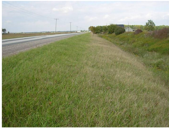
Figure 12.1 Roadside vegetated filter strip (TWG 2008)
