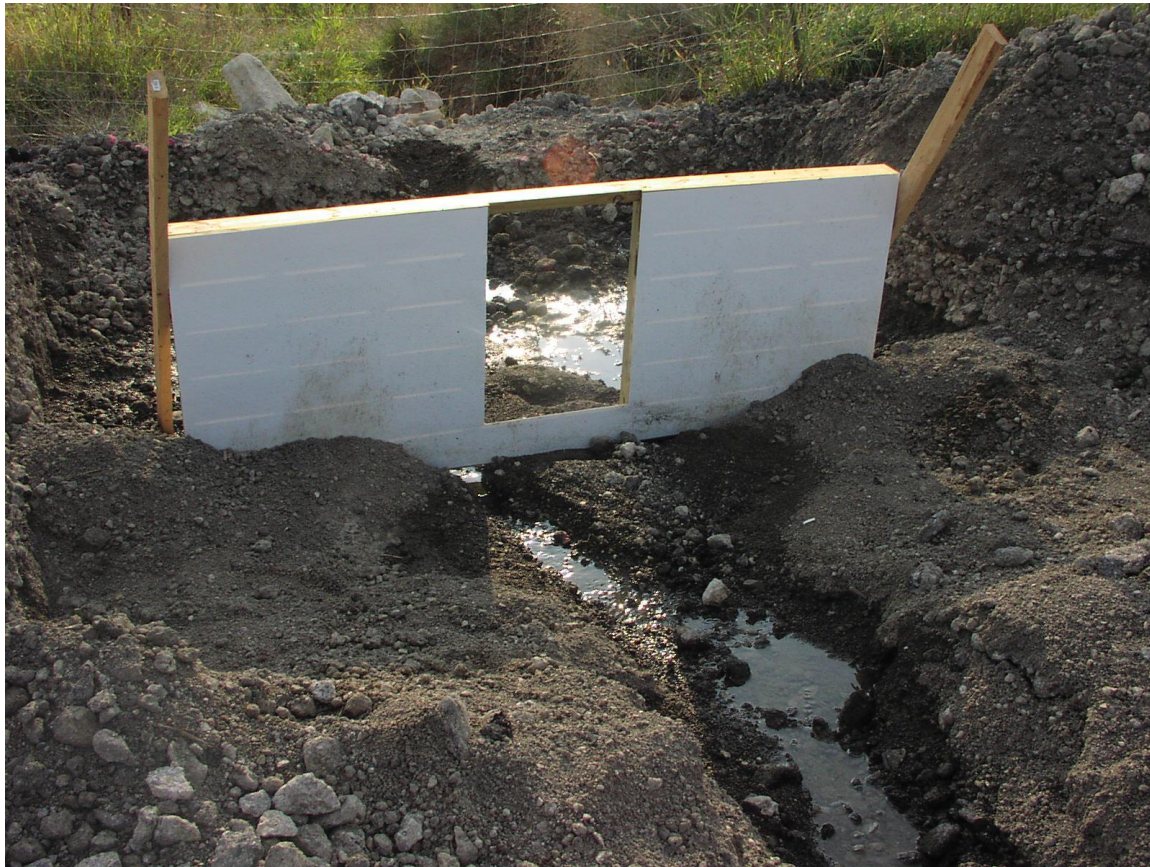
Figure 4.3 Rectangular weir installed at site A
