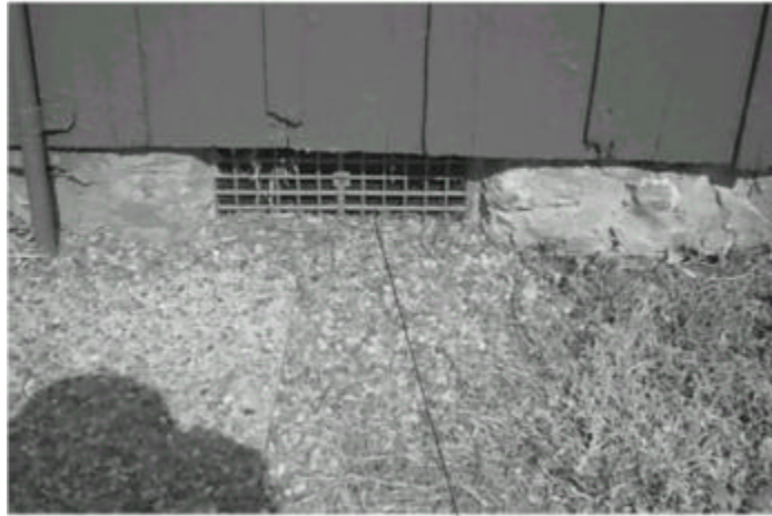
Crawl space vent properly screened
