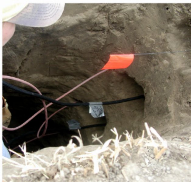
Figure 4. TDR probes and soil thermocouples installed in the field.
