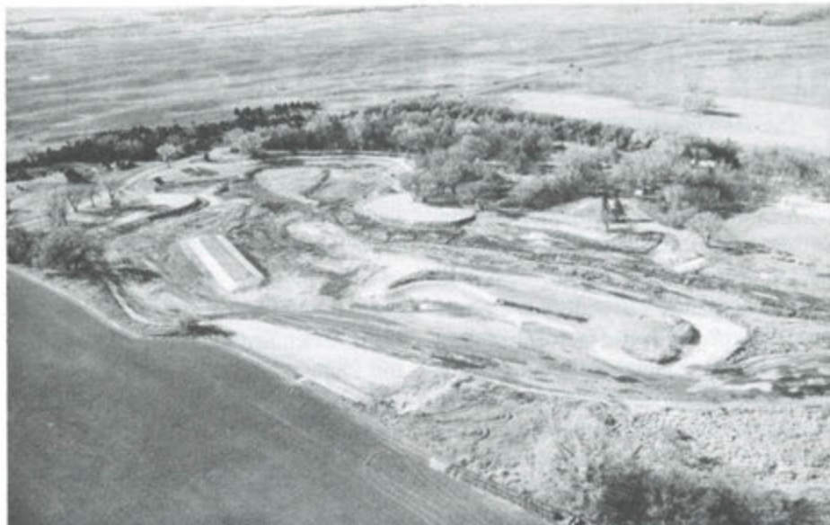
Aerial view of Pibel Lake during rehabilitation.
