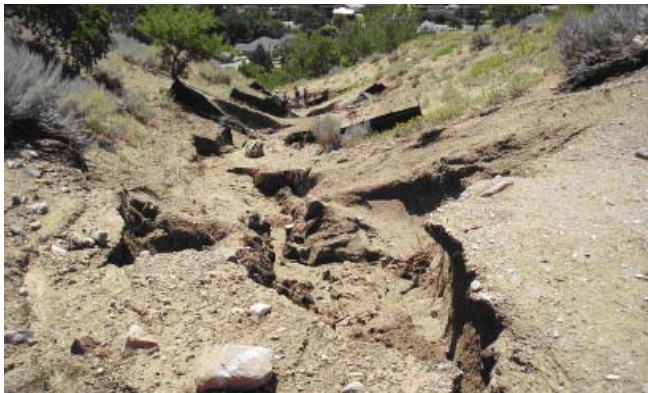
Most often silt fences are destroyed during a debris flow that rips through the center of a channel.
