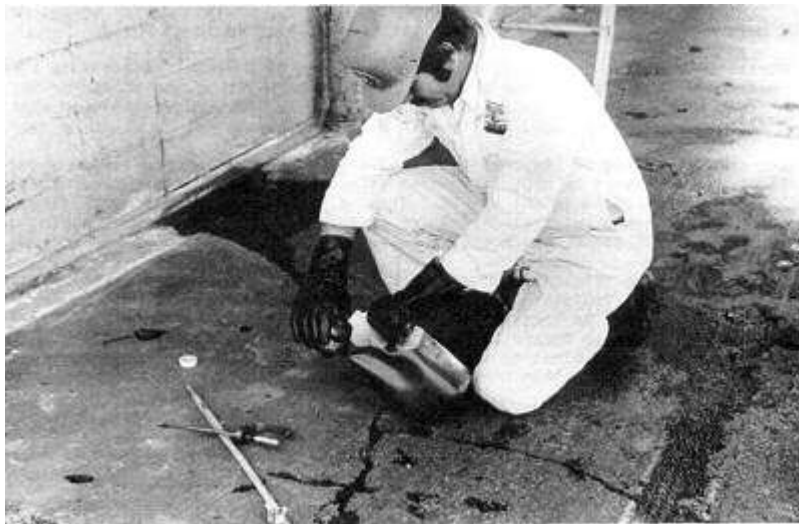
FIGURE 4. Filling trigger oil can with Rid-A-Bird solution. The service technician is wearing protective gloves as well as coveralls and hard hat.
