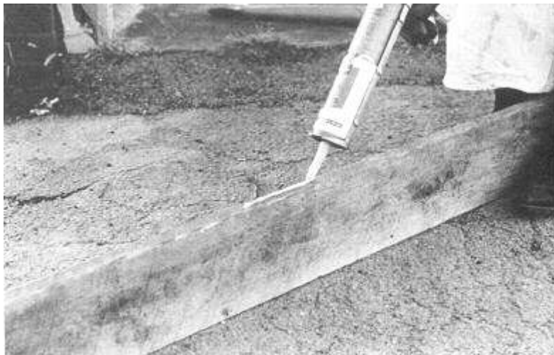
FIGURE 2. Apply repellent past 1/2" back from the edge of the ledge. The strip of repellent paste should be 1/4" wide and 1/4" high.
