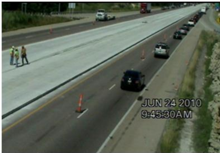
Figure 3.1 Work Zone View from a Data Collection Camera, Interchange at Mile Marker 253, I-44 WB
