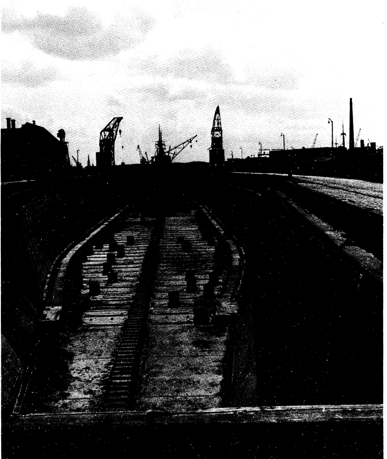
Figure H-7. Graving dock.
