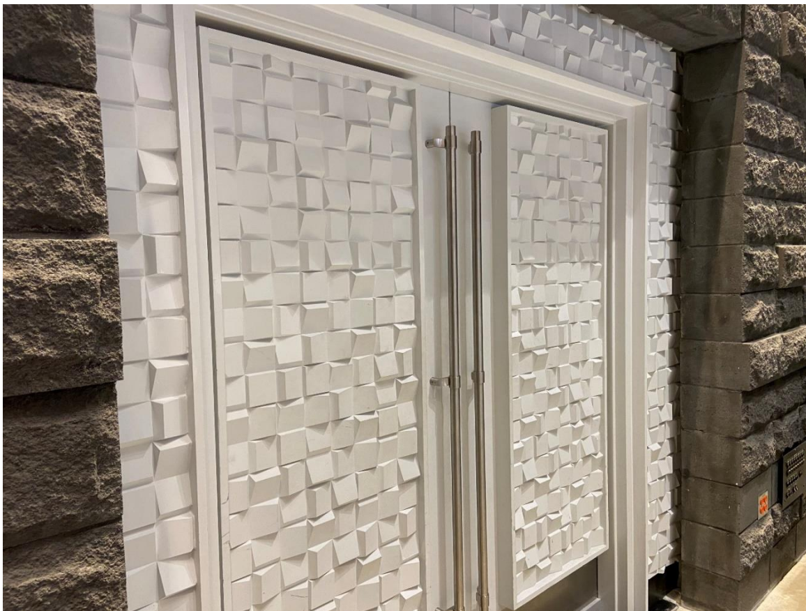
Figure 3.7: Example of a surface designed to augment a room's sound scattering properties; photograph taken in the Strauss Performing Arts Center recital hall
