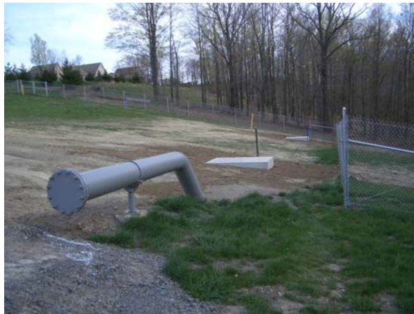
Figure 1. Access points for 12" Cased Pipe
