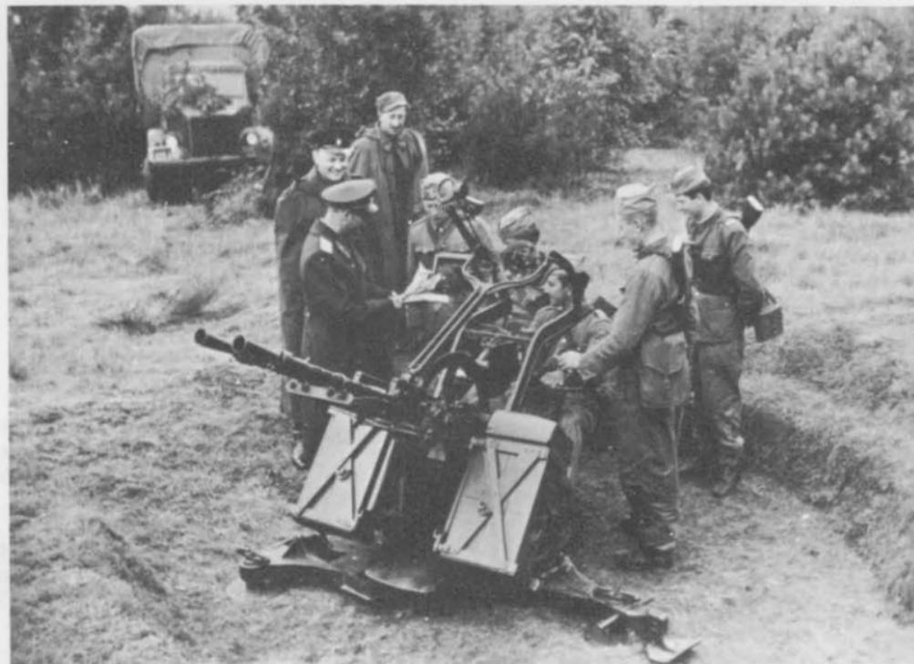
SOVIET 14.5-MM TWIN AA MACHINE GUN, ZPU-2.
