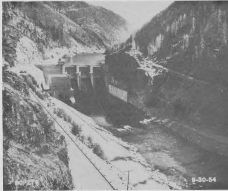
Figure 109: Tainter Gates Scale Unknown
