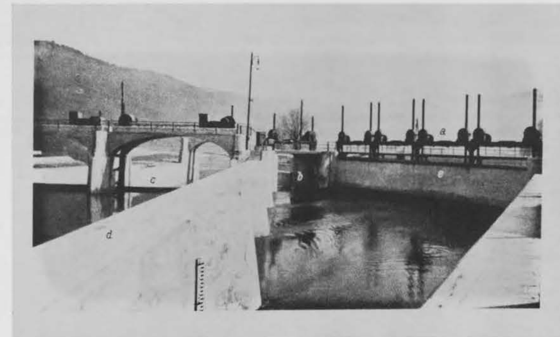
Figure 98: Canal Intake Structure
