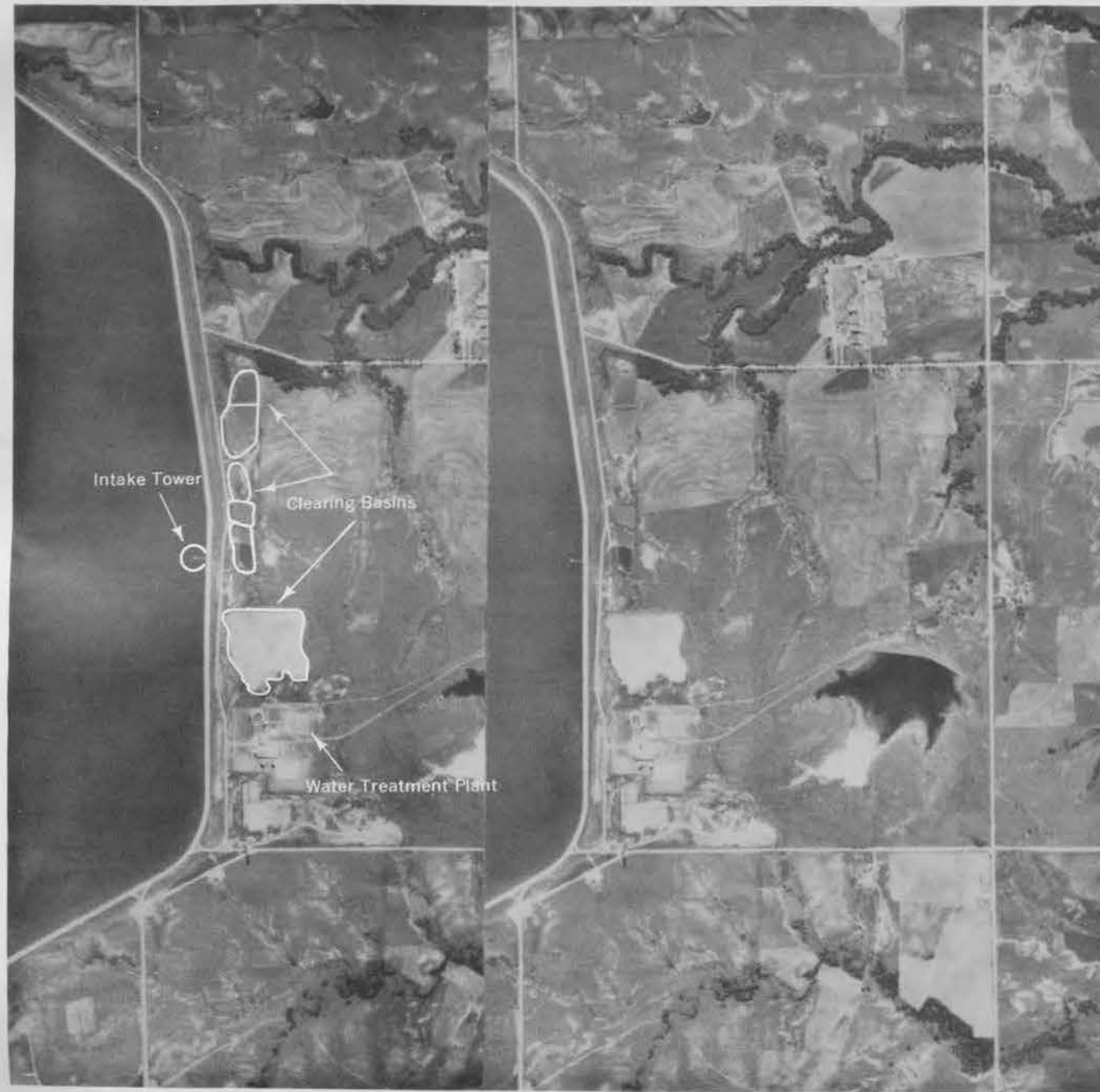
Figure 96: Water Supply Intake Scale Unknown
