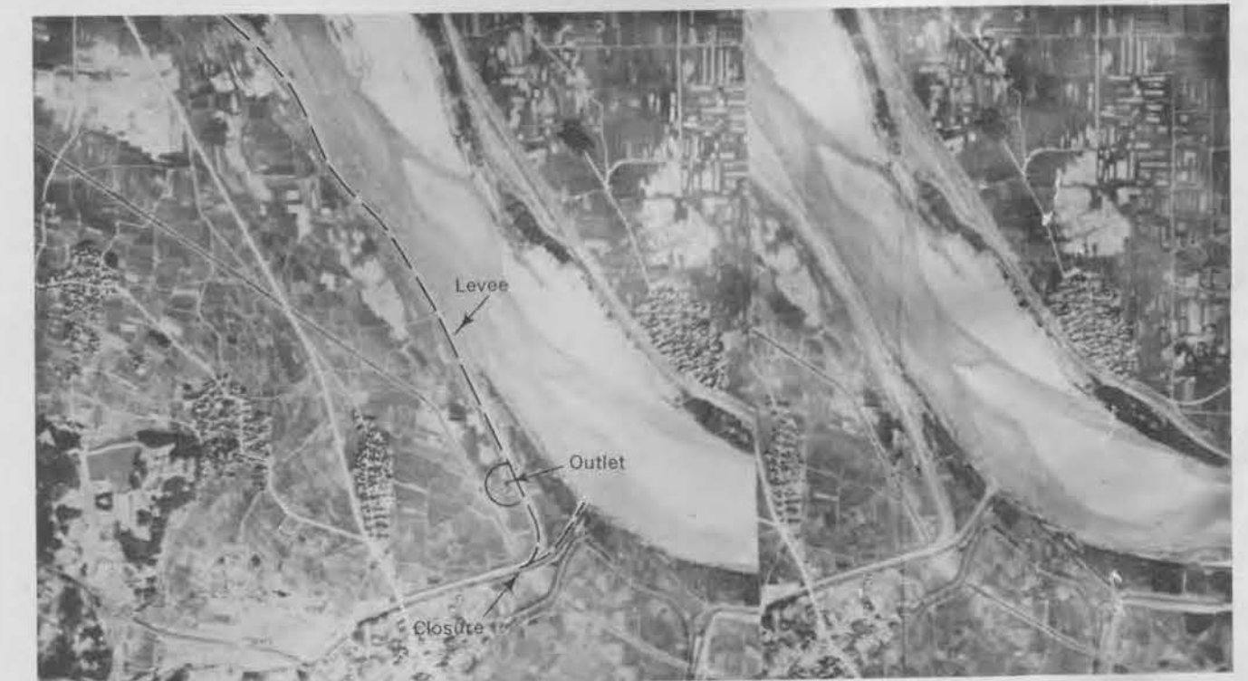
Figure 128: Open Levee Scale Unknown
