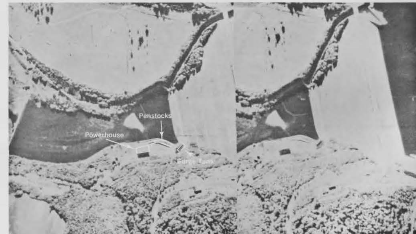
Figure 100: Penstocks Emerging from Dam Abutment Scale Unknown
