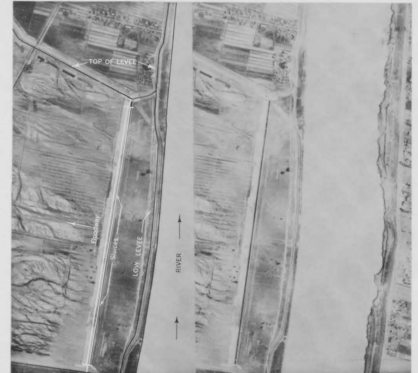
Figure 134: Floodway Diversion Works Scale Unknown
