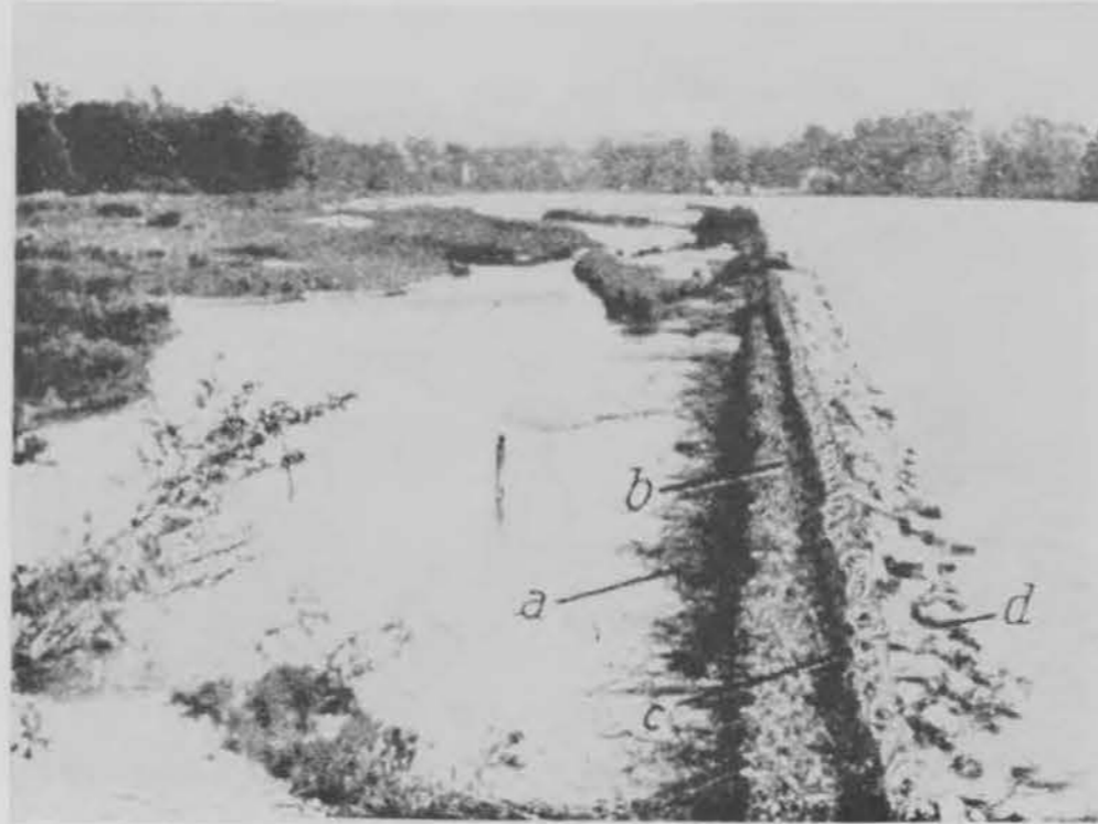
Figure 135: Training Wall without Traverses
