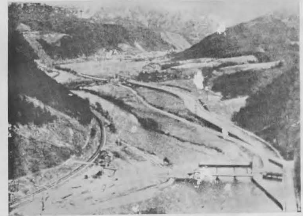
Figure 101: Diversion Canal (Hydropower)
