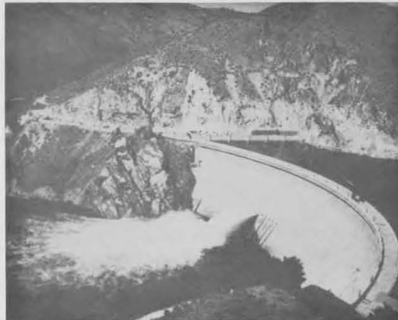
Figure 116: Sluice Outlets, Masonry Dam
