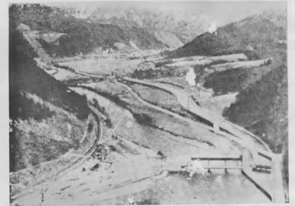
Figure 101: Diversion Canal (Hydropower)
