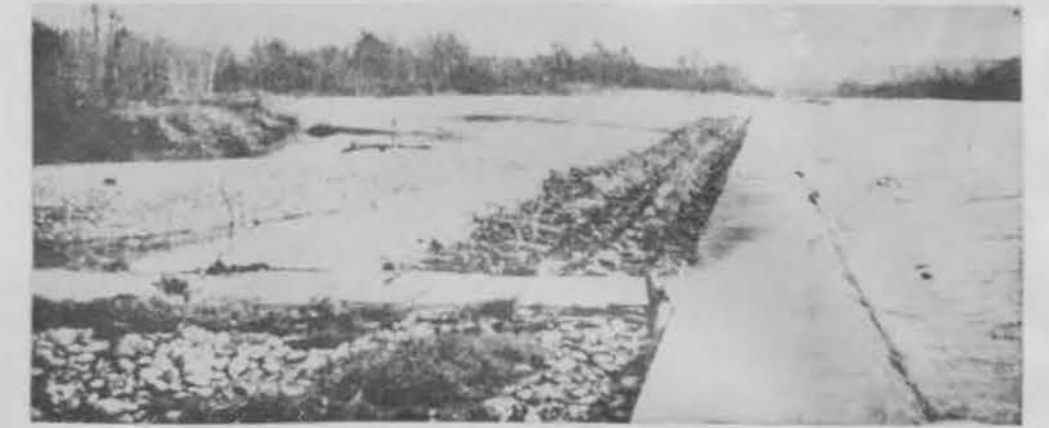
Figure 137: Training Wall with Traverse
