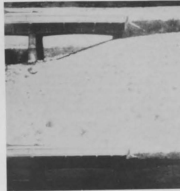
Figure 142: Dumped Riprap
