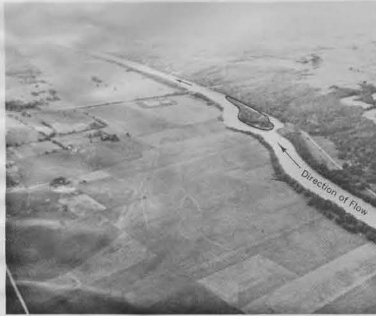
Figure 65: Island The blunt end of the island is upstream.
