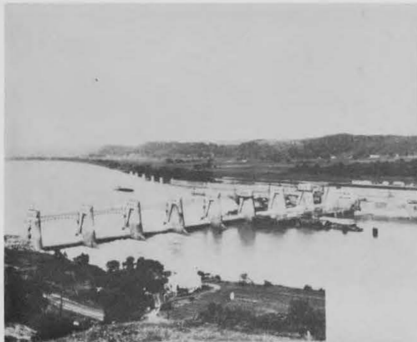
Figure 110: Roller Gates Scale Unknown
