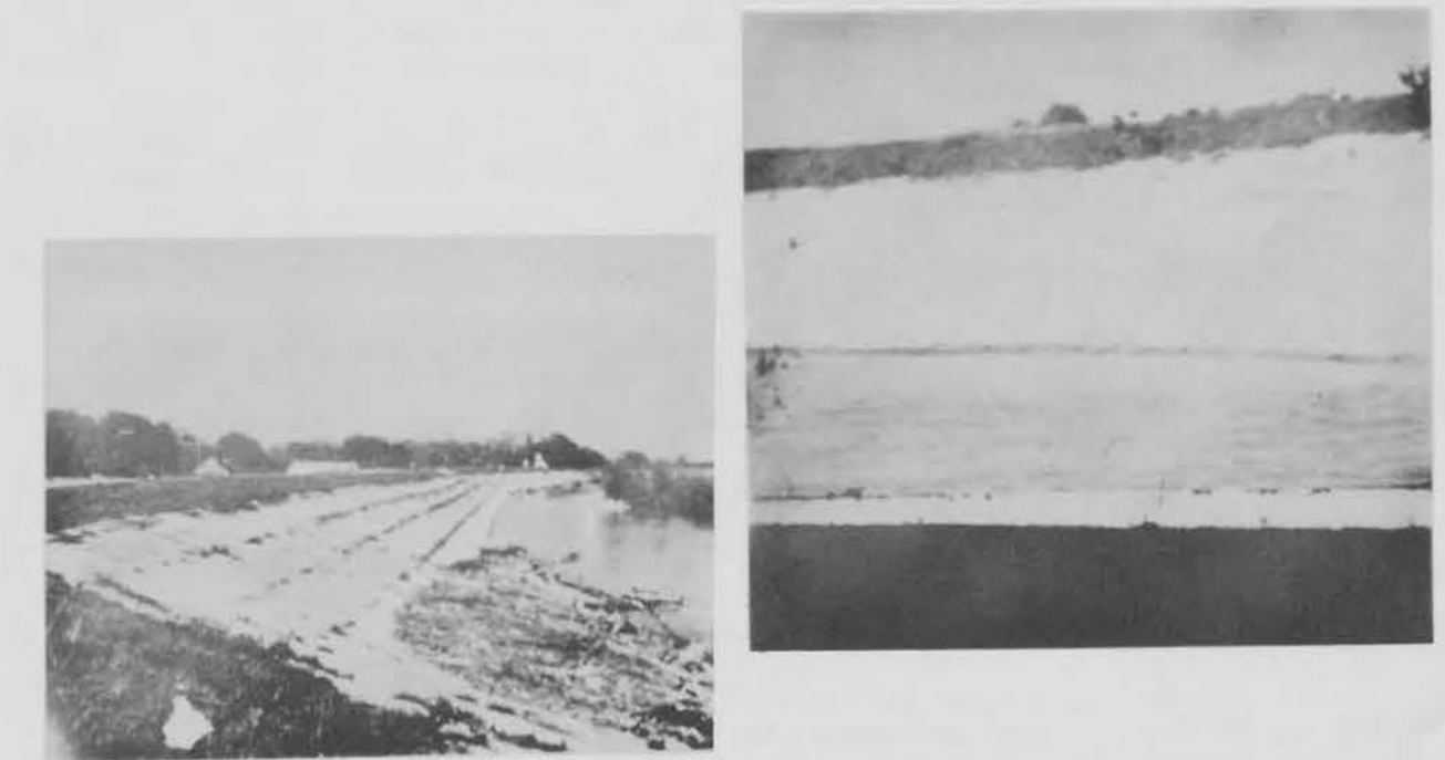
Figure 145: Articulated Concrete Mats
