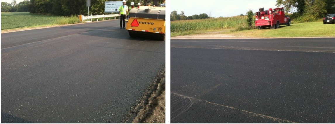
Figure 3.8 The construction process of the intermediate layer
