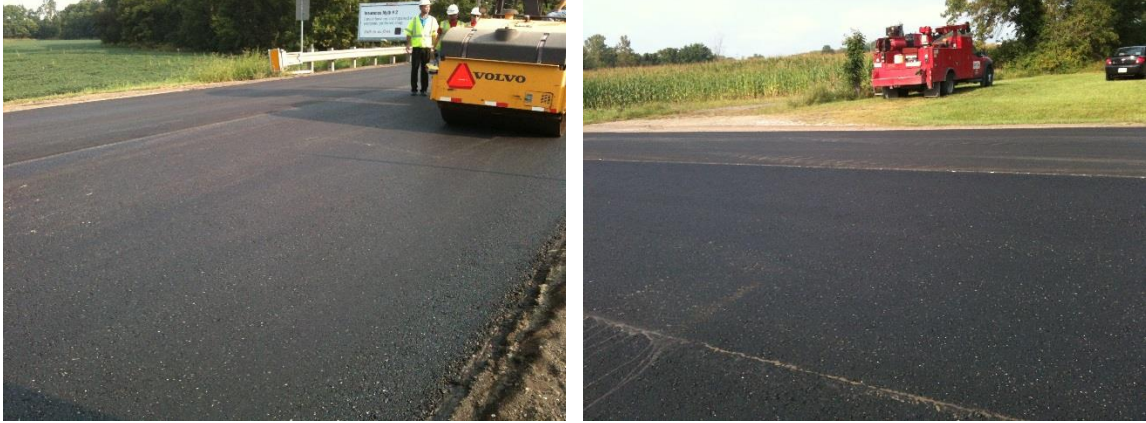
Figure 3.8 The construction process of the intermediate layer
