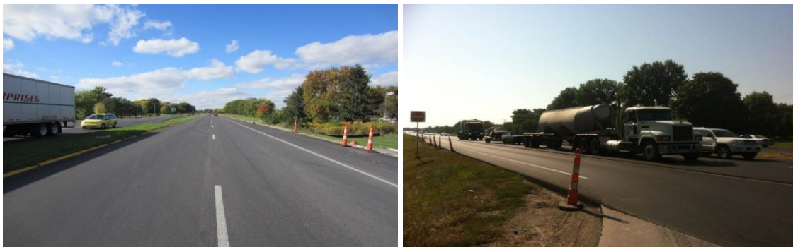
Figure 3.4 Test sections after compaction
