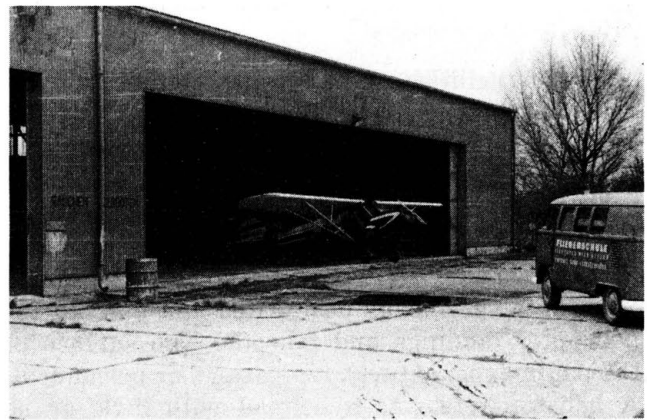
Figure 5-60. Hangars and hardstand at light aircraft airfield.
