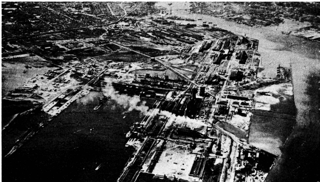
Figure 7-8. Iron and steel plant.
