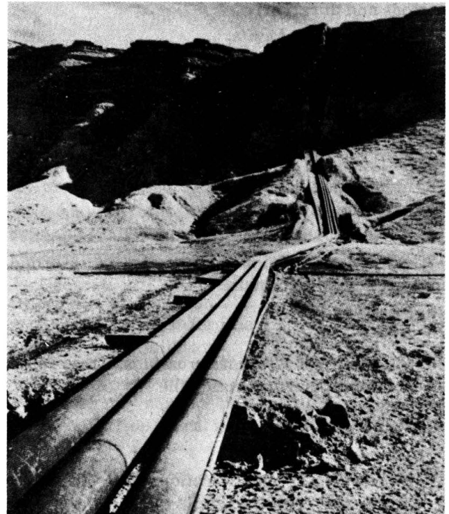
Figure 5-20. Pipeline laid above ground.
