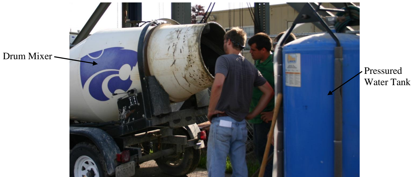
Figure 3.8 Adding Water to Mixer
