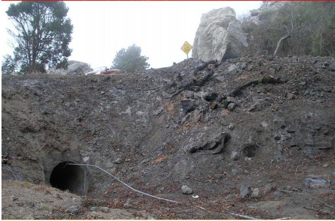
The consequences of a major wildfire can be far reaching. This photo shows a culvert near Big Sur, California, which could be blocked by a landslide or debris flow, closing a major highway for several days.
