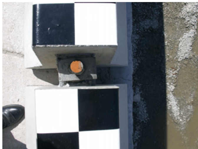
Figure 9. Barrier Connection Joints
