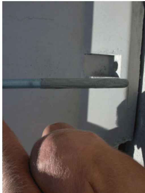
Figure 11. Barrier Tie-Down Installation
