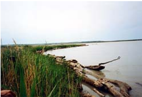
Figure 1. An Army Corps (WES) stabilization project using logs cabled in place and revegetation planted on bankline. Lake Sharpe, South Dakota, June 1994.
