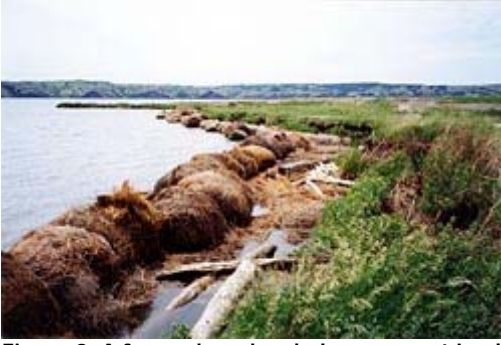
Figure 3. A farm where hay bales were put in place Sept/Oct of 1993. Note the height of the vertical cutbanks in the background, which are common to the entire lake. Lake Sharpe, South Dakota, June, 1994.
