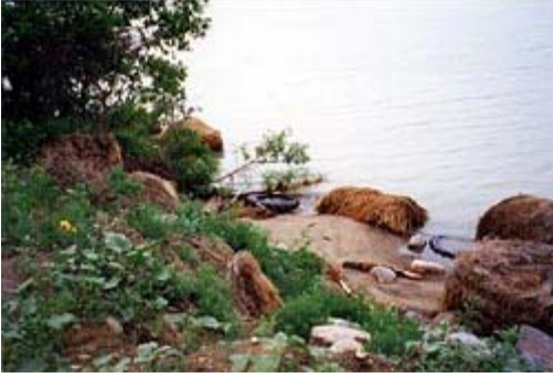
Figure 6. A stabilization at the Fort George Game & Fish Commission (with no Army Corps involvement) attempted to use tractor tires and hay bales. Note the sand buildup behind the center bale. Lake Sharpe, South Dakota, June, 1994.
