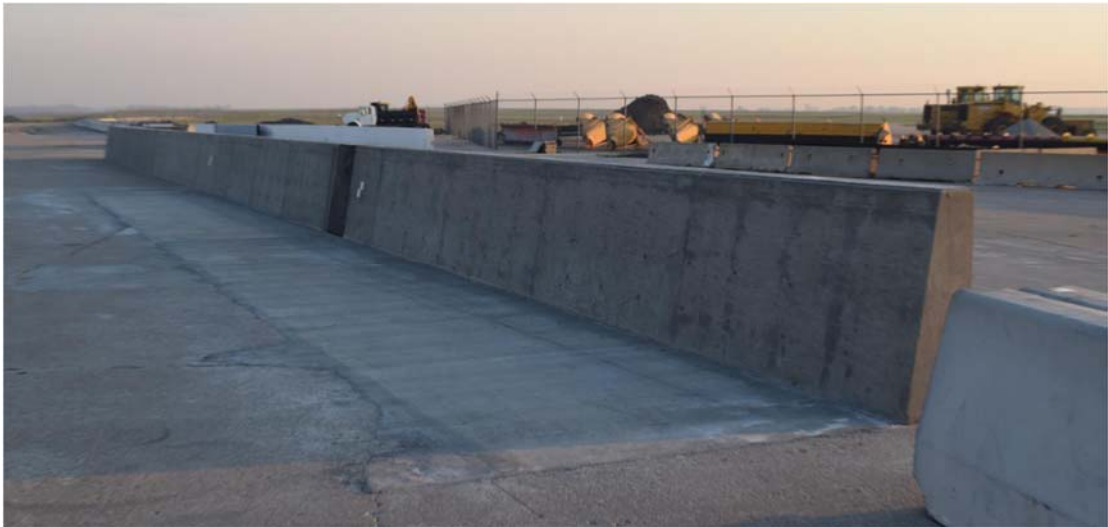
Figure 2: Test installation photographs
