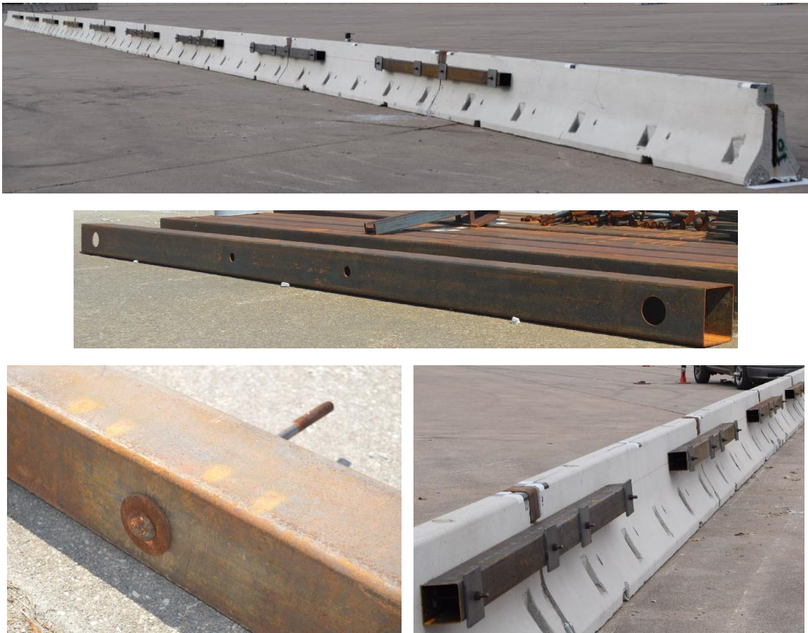
Figure 13. Box Beam Stiffeners
