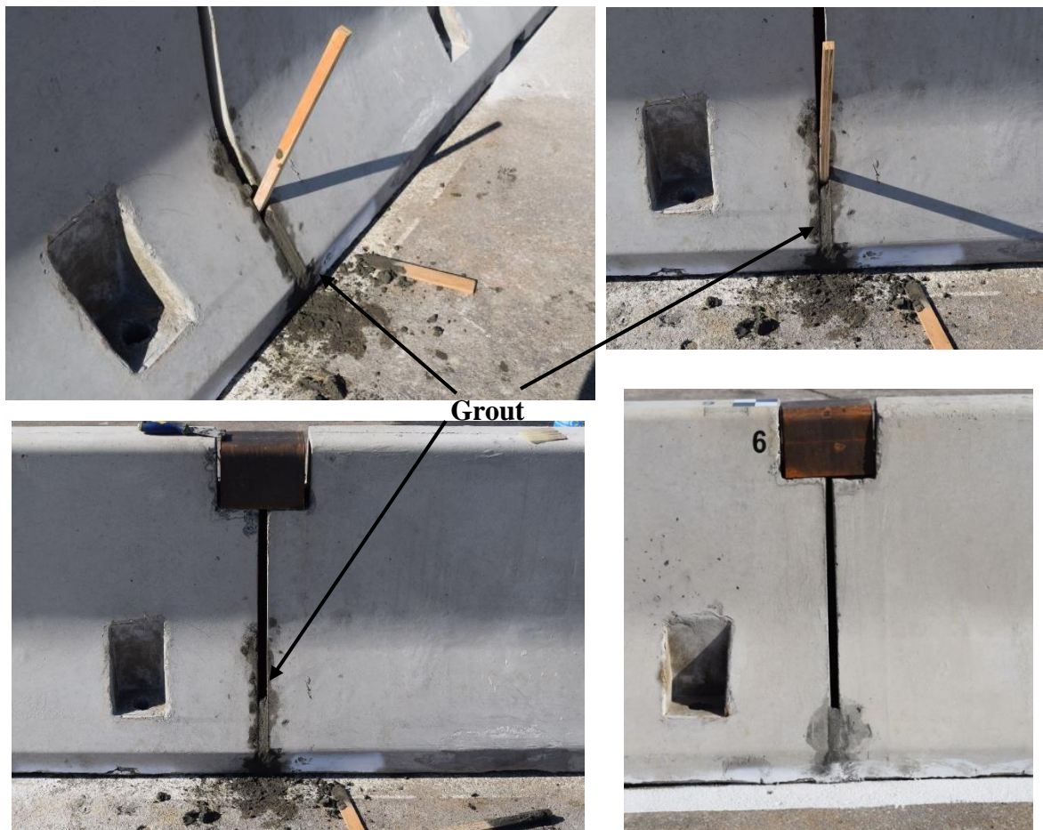
Figure 14. Non-Shrink Grout between barriers
