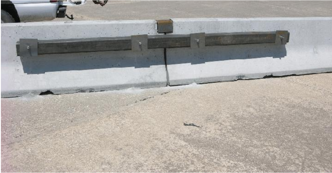
Figure 2. PCBs with Box-Beam Stiffener
