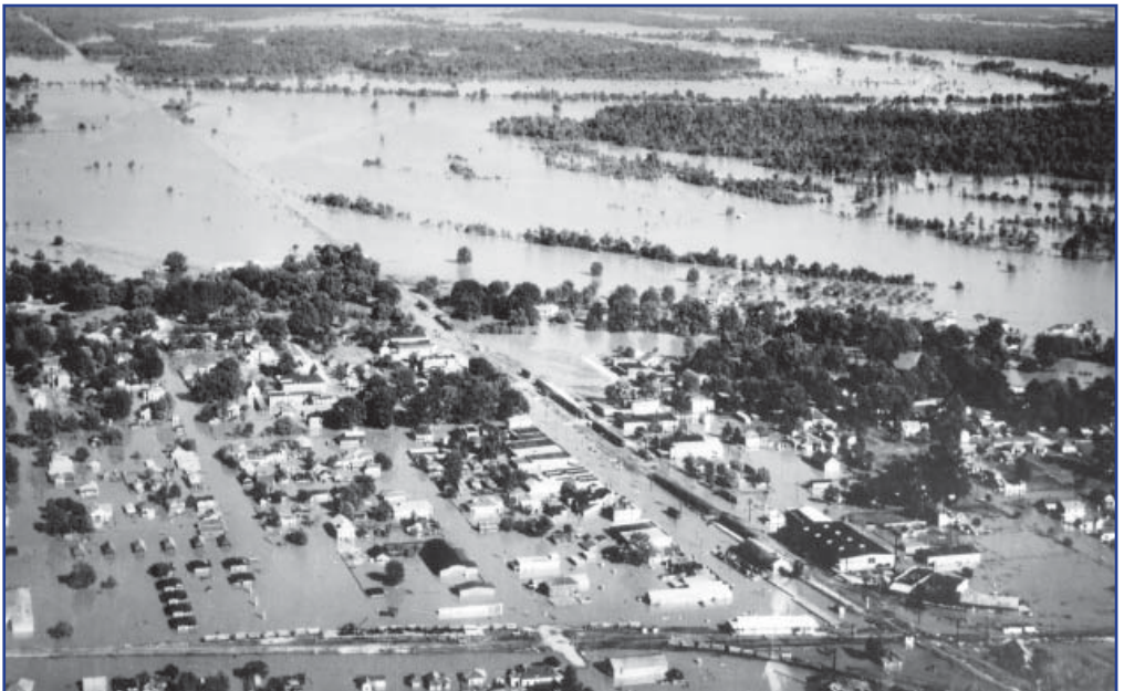
Floodwaters inundate Tallulah, La., after the Cabin Teele levee crevasse.
