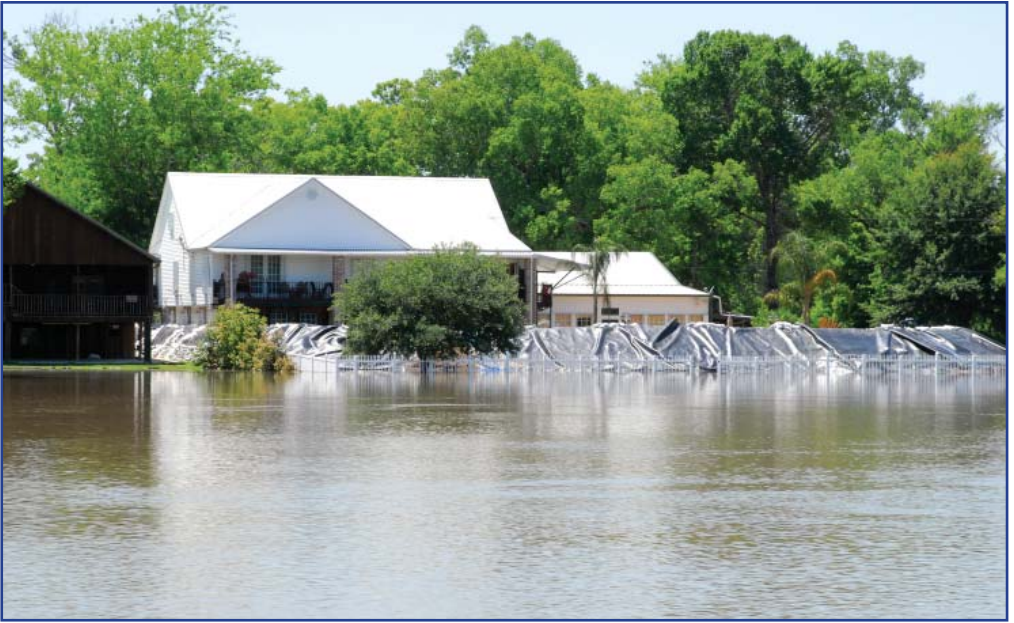
An example of “flood proofing” in the Atchafalaya basin.
