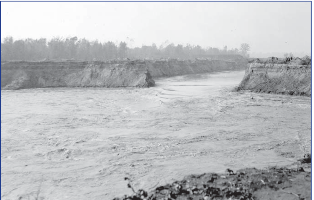
One hour after opening, erosion of the plug has spread.
