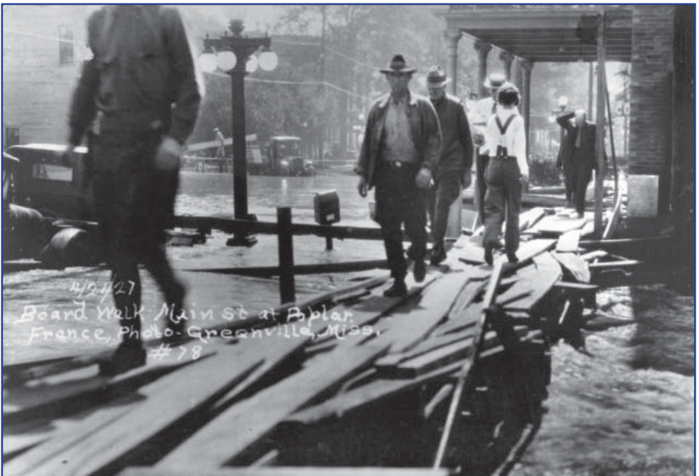
Greenville, Miss., after the Mound Landing levee crevasse.
