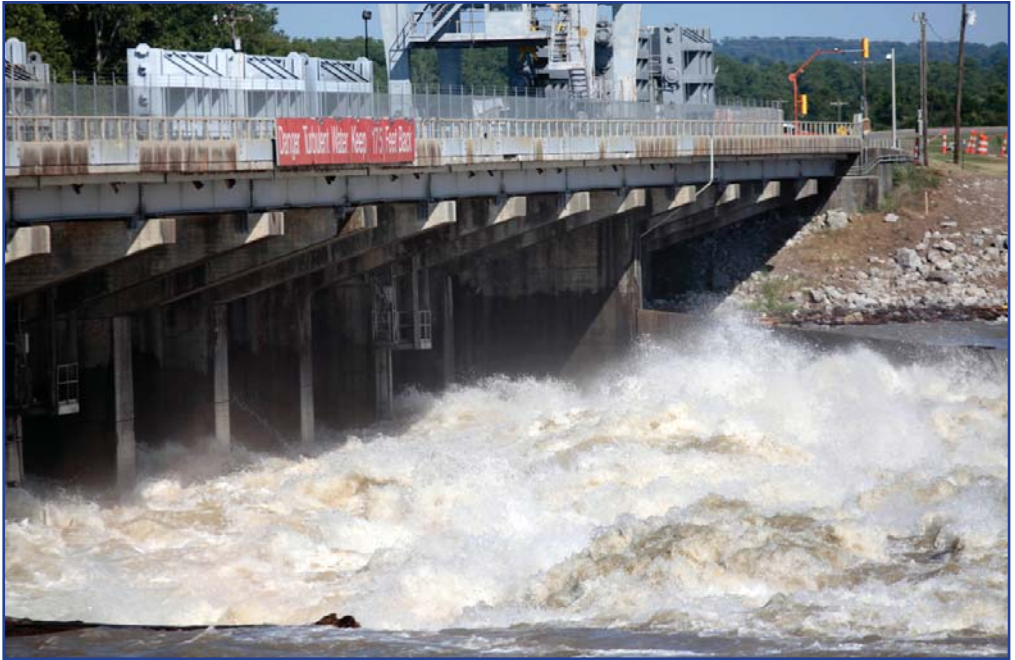
The Low Sill Structure at the Old River Control Complex on May 14, 2011.
