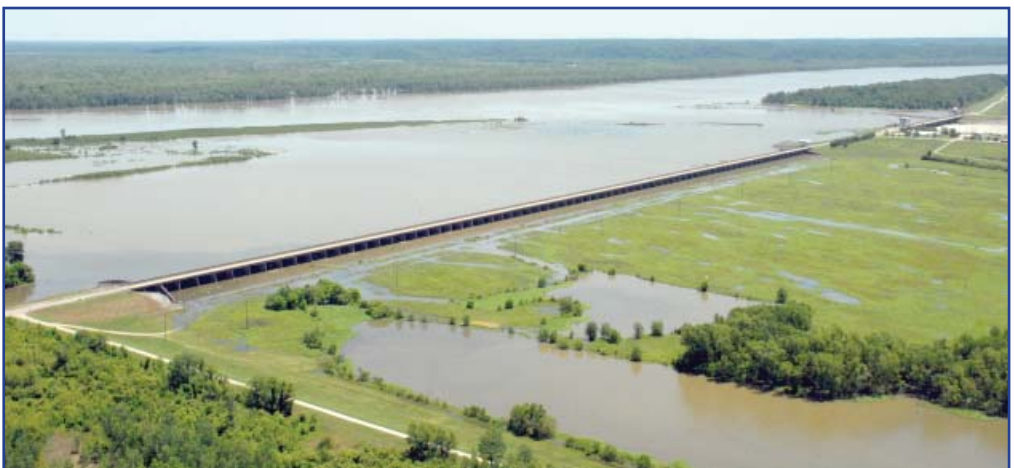
Water seeps through the overbank structure at the Old River Control Complex on May 4, 2011.
