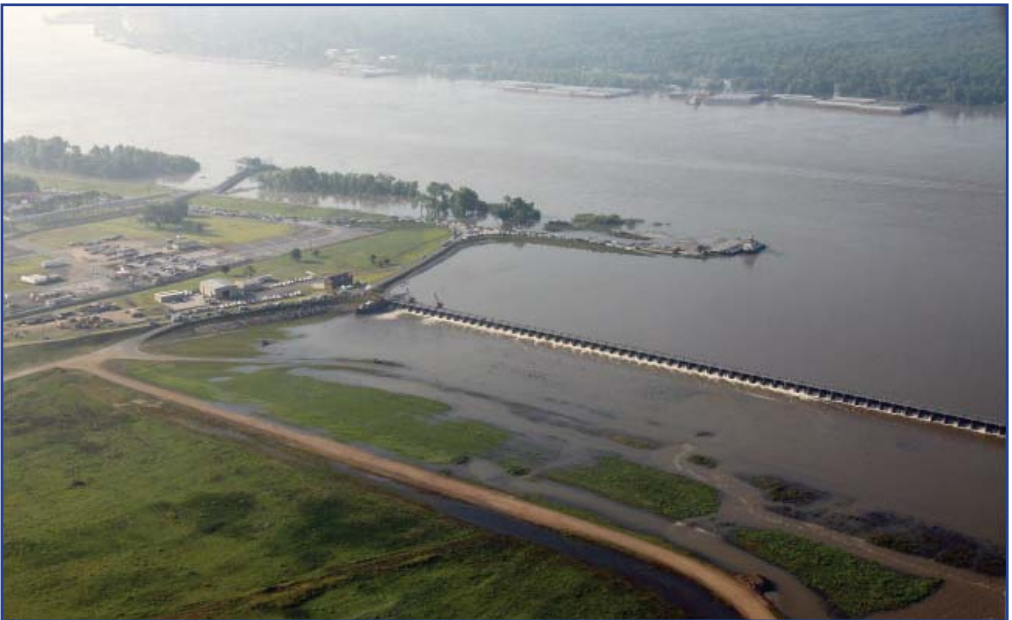
Aerial view of the Bonnet Carré floodway just moments after the spillway was opened.
