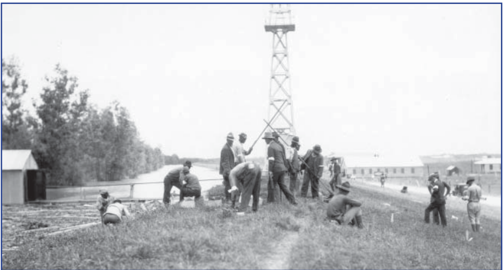
Workers prepare the Caernarvon levee crevasse site. (Library of Congress)
