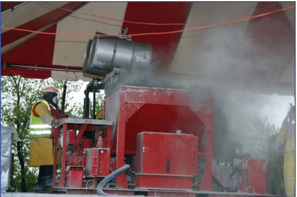
Members of the floodway task force prepare the explosive slurry mix.
