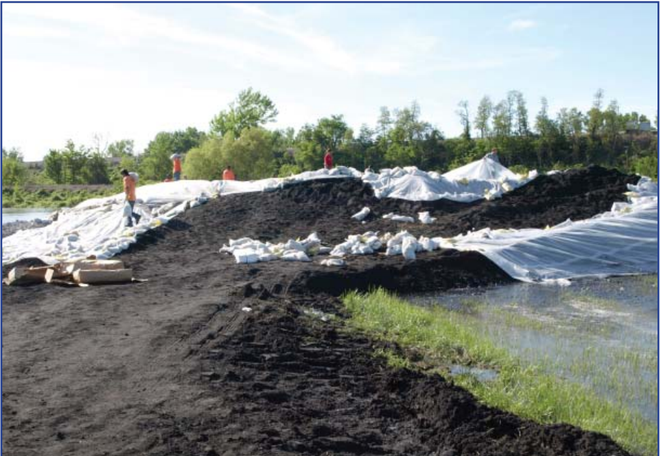
Below: The flyash cinder ring berm at the Cairo mega boil.
