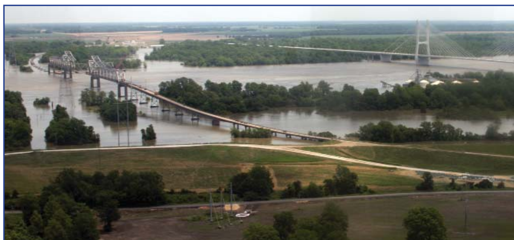
White sand boil rings near the toe of the levee at the Greenville bridge in Arkansas.
