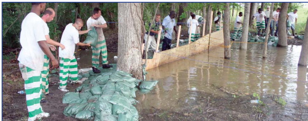
Levee workers and inmates address the high energy boil at Winterville.
