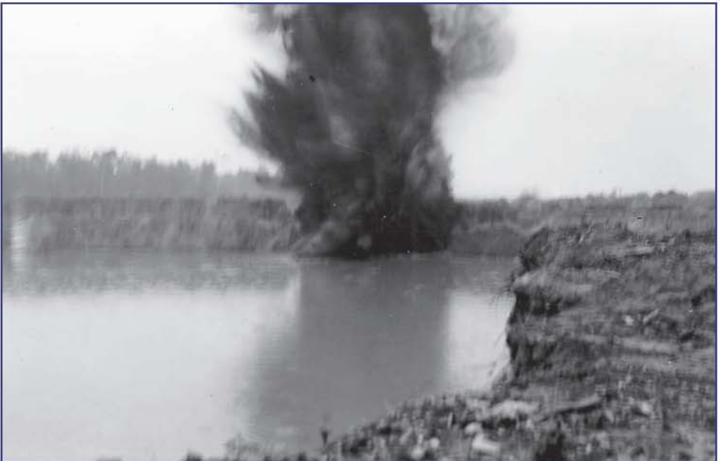
Dynamite removes the plug and opens the cutoff.
