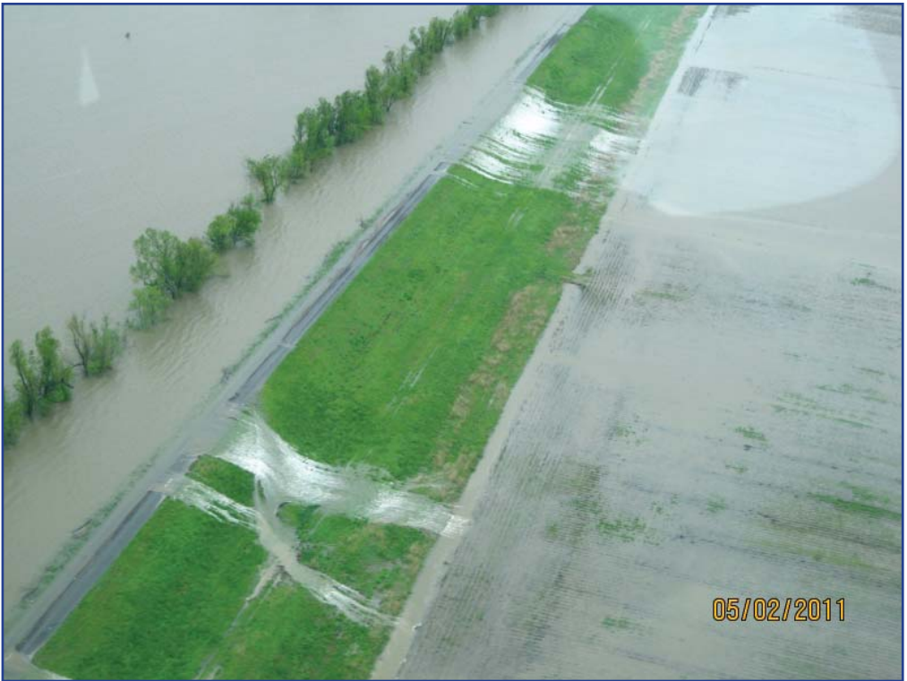
Passive activation of the floodway. The Mississippi River overtops the lower sections of the Birds Point-New Madrid floodway fuseplug levee early on May 2, 2011.
