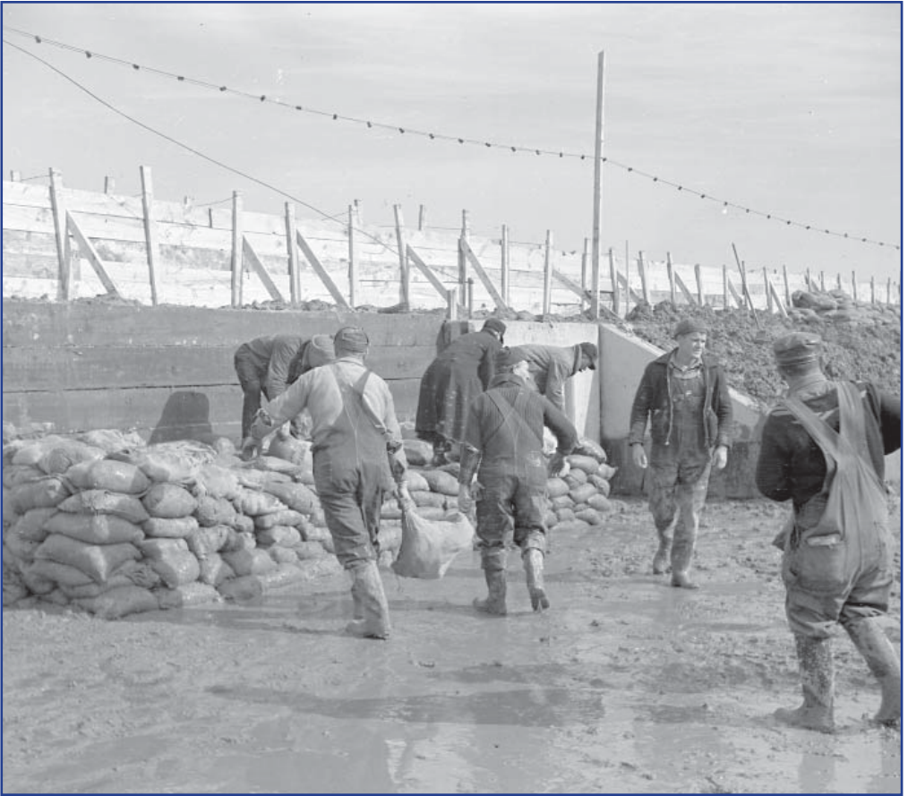
Workers raise the level of protection at the Cairo floodwall during the 1937 flood. (Farm Security Administration - Office of War Information Photograph Collection, Library of Congress)
