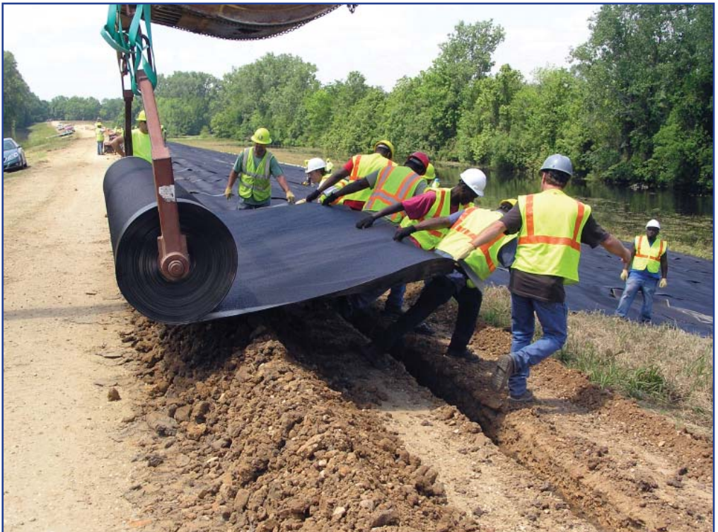
Armoring the Yazoo backwater levee.
