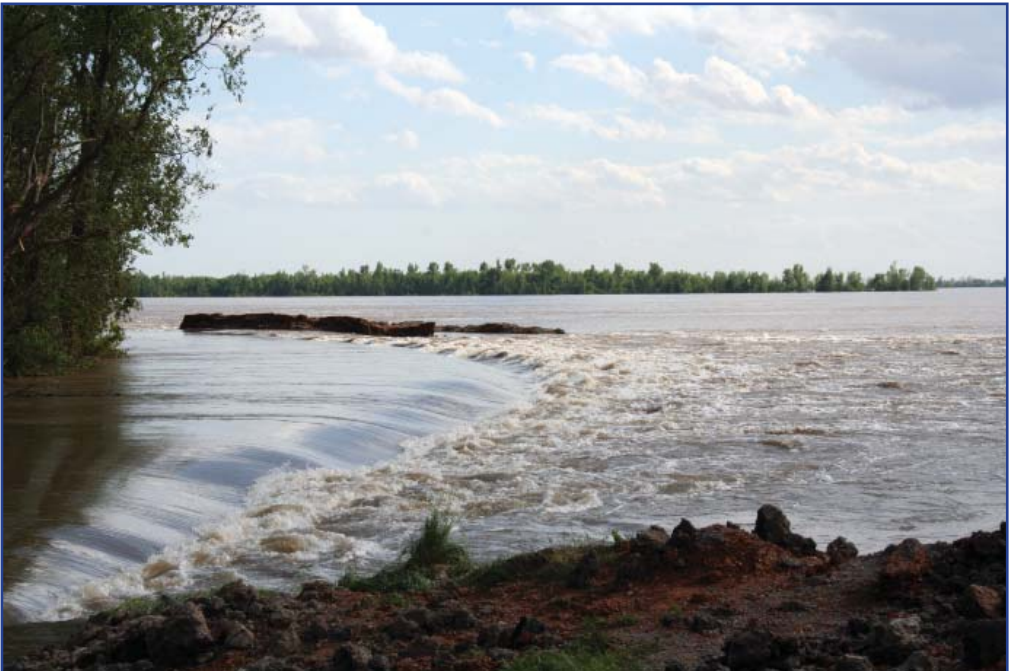
Water roars through the upper inflow crevasse at the frontline levee the day after activation.
