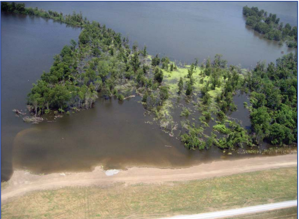
Water from Eagle Lake creates a water berm over the earthen berm at Buck Chute. Note the outline of the earthen berm under the water.
