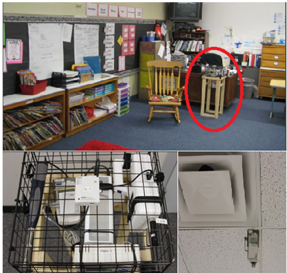
Figure 1. Equipment housing placed next to teacher's desk (photo on the top), close looking of the special housing (photo at the lower left), hanging CO 2 m (photo at the lower right) [8].
