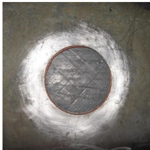
Fig. 2 Mounted concrete slab at test port viewed from inside RF shelter
