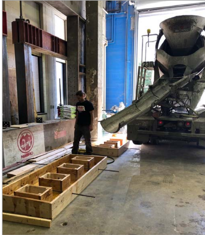
Figure 5-2. Concrete placement
