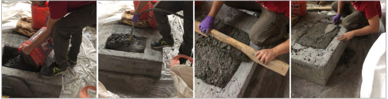
Figure 5-5. Slab patching process
