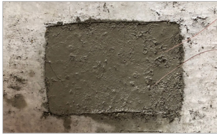
Figure 5-6. Finished patch surface
