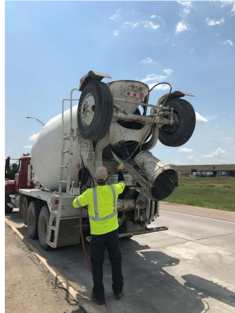
Figure 2-2. Typical process of chemical admixtures being prepared and introduced into a mixing truck at the job site
